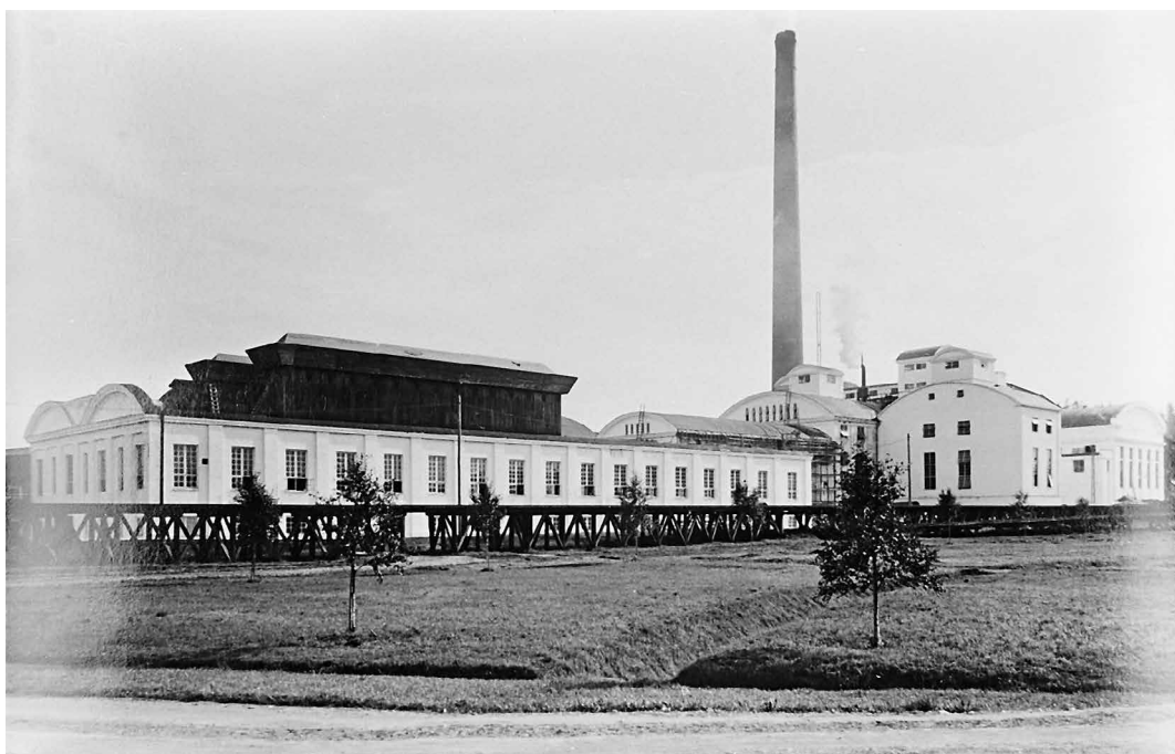
The Diesén Wood Pulp Mill in Pitkäranta in the 1930s. Photo: The Finnish Heritage Agency, Helsinki, Finland. CC BY 4.0.
