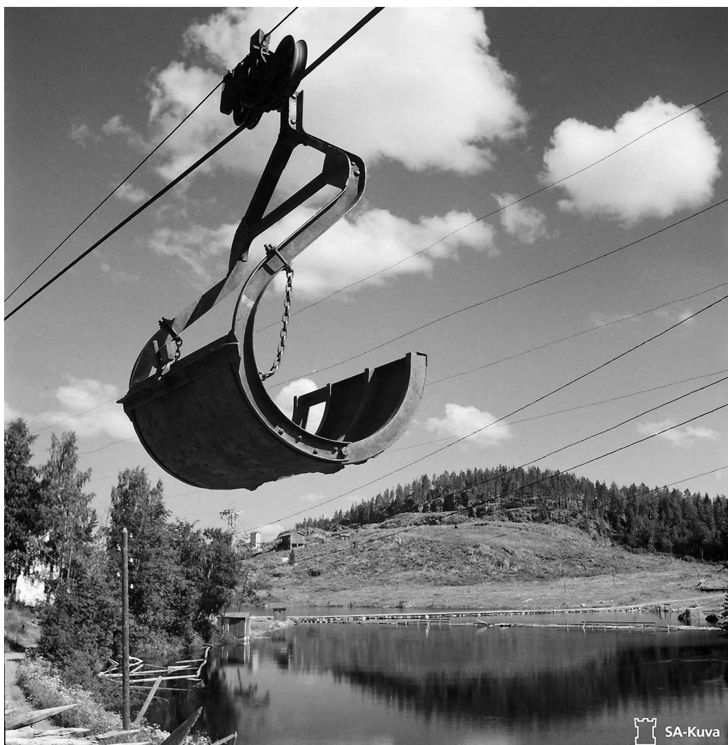
The aerial tramway/téléphérique of the Leppäkoski pulp mill by the Jänisjoki river. The broad clearcutting riverbank is visible in the background. Photo: SA-Kuva 1944, Finland. CC BY 4.0.
