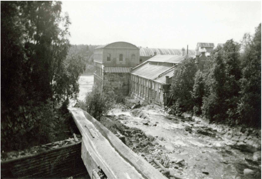
The log flume of the Läskele paper mill. Photo: O. Varsta 1939. Forest Museum of Lusto, Finland. CC BY 4.0.
