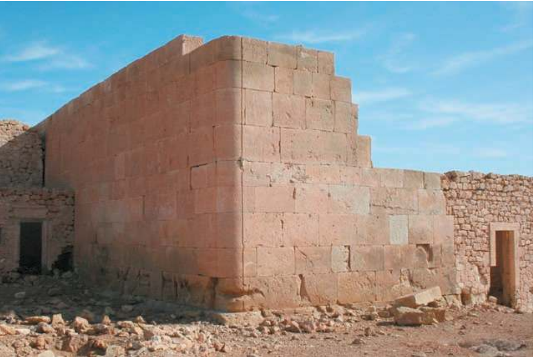
Fig. 108. The fine masonry of the Roman fortlet at Qaryah Ash-Sharqiyah stands out from its enveloping Italian successor.
