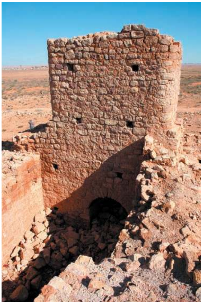
Fig. 109. Qasr Wamis: the tower above the entrance, seen from the inside.
