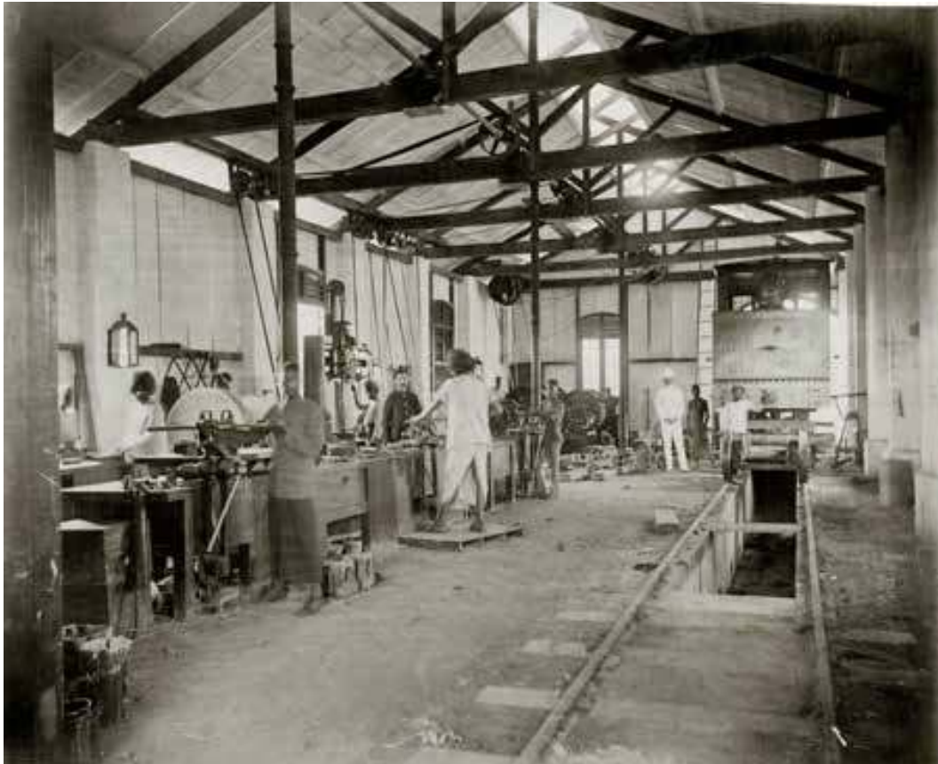
Figure 2.2. Railway workshop, 1880s–1890s. © Colonial Office, Commonwealth and Foreign and Commonwealth Offices, Empire Marketing Board, and related bodies. Courtesy of the National Archives, United Kingdom, used with permission
