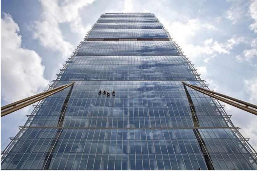
Fig. 8.1 Allianz Tower while human workers are cleaning the façade. (Credit: Piermario Ruggeri-Focchi façade)
