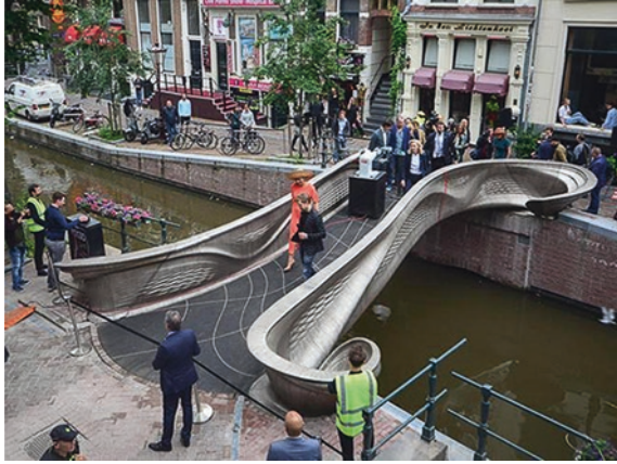
Fig. 8.3 MX3D Bridge. (Photo by Adriaan de Groot)
