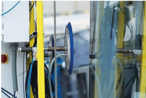
Fig. 8.9 Hephaestus details during façade installation. (Credit Alex Iturralde)
