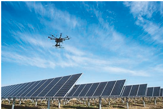
Fig. 8.6 Thermography inspection of a PV plant by drone
