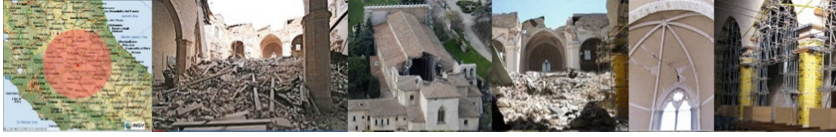
Fig. 1. The area struck by the earthquake at L'Aquila and the damaged Basilica di Collemaggio
