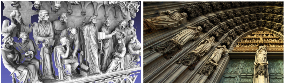
Fig. 9. Shadow effect on the survey data by staggered surfaces (tympanum and jamb figures at Cologne Cathedral, west portal) and with filled gaps 2 .
