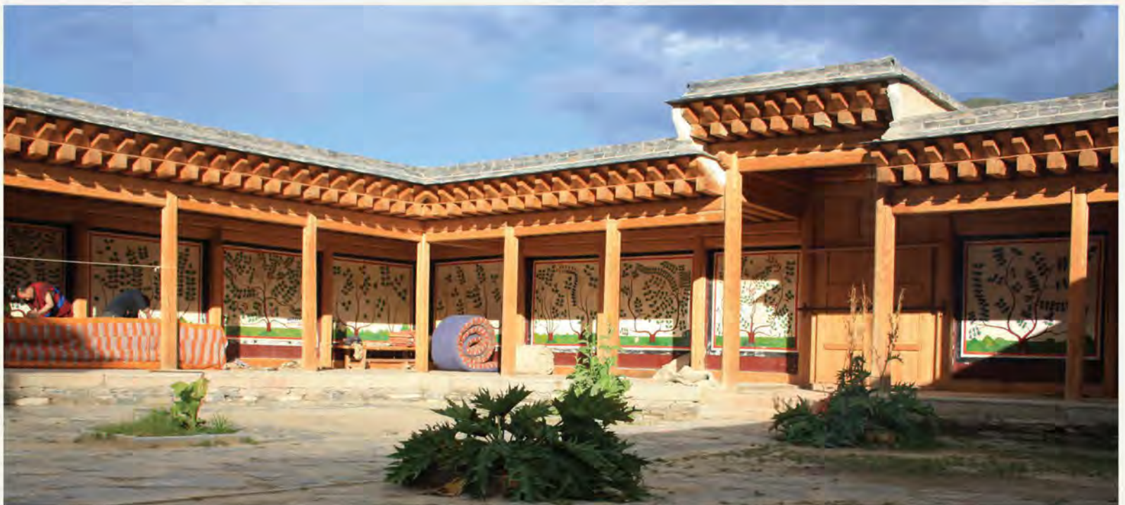
V2.1 Tree Murals in the Inner Courtyard of the Medical College at Labrang Monastery after a recent renovation
