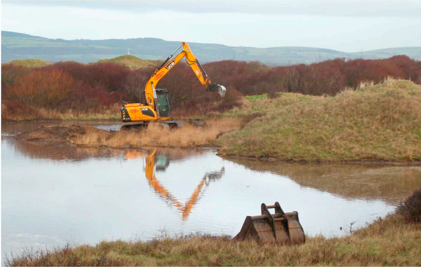
Figure 16.13 The dune slack excavations took place in winter, often while the slacks were under water. The stand of Molinia in front of the excavator shows the habitat structure before the excavation work started.
