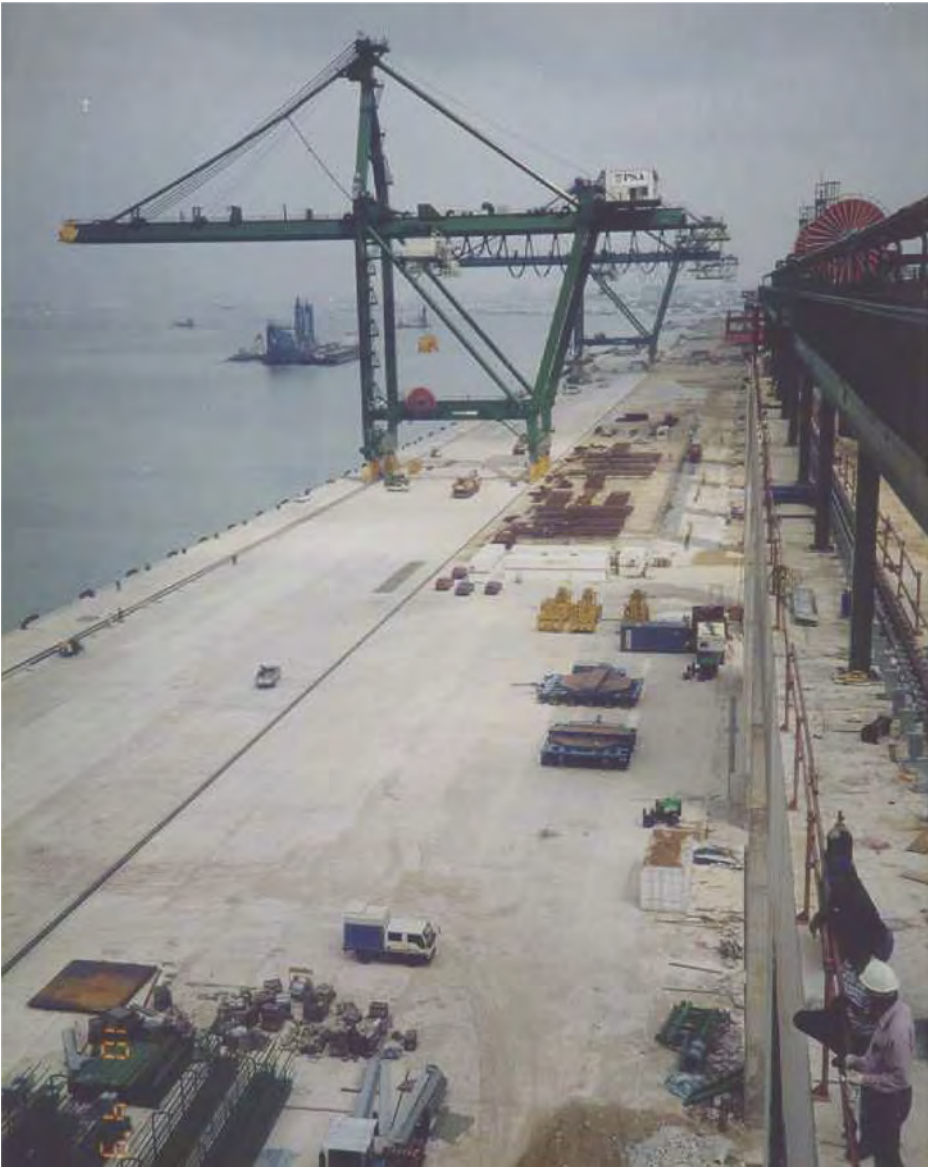
Figure 2. Singapore Pasir Panjang Container Port Phase 1 wharf front after completion.
