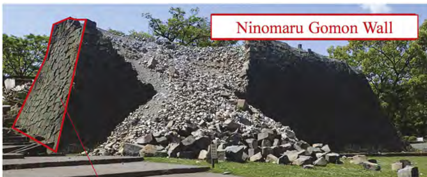
Figure 1. Collapsed masonry wall of Kumamoto Castle during the 2016 Kumamoto Earthquake (Kamiya et al., 2018).
