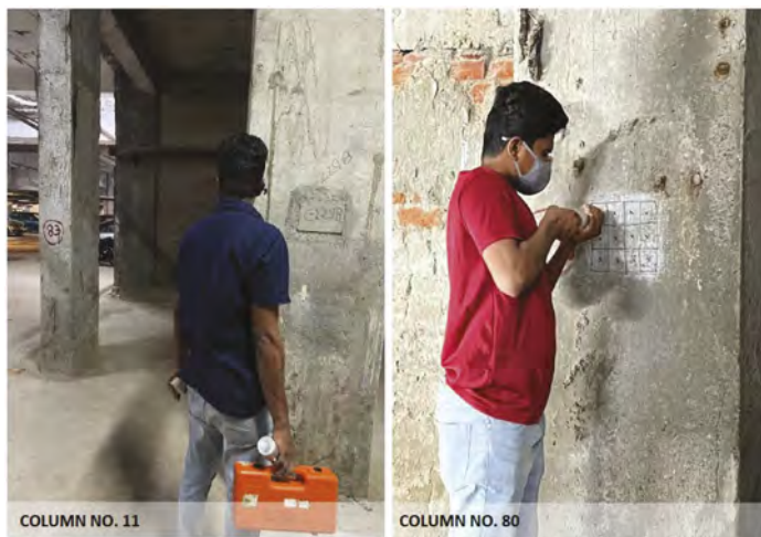
Figure 7. Conducting NDT tests at Aster 2.
