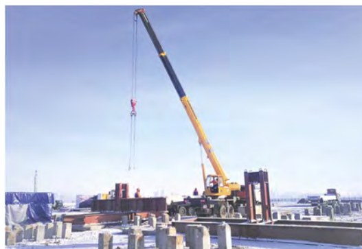
Figure 1. Mounting kentledge system.
