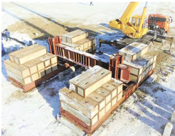
Figure 2. Assembling loads during mounting kentledge system.
