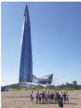
Figure 1. General view of Lakhta center multifunctional complex.
