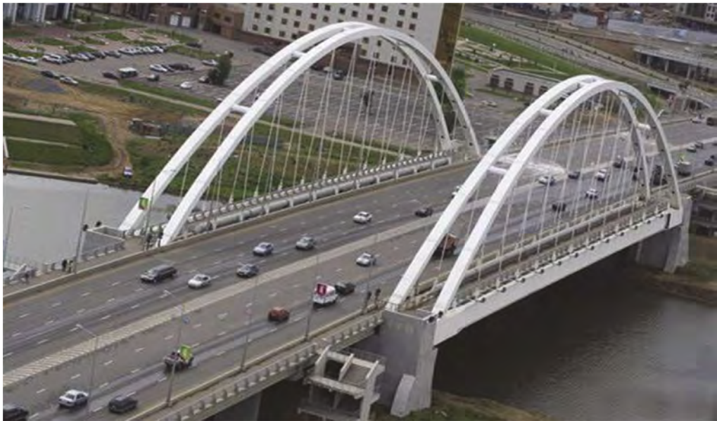
Figure 1. “Argali” bridge in Astana.
