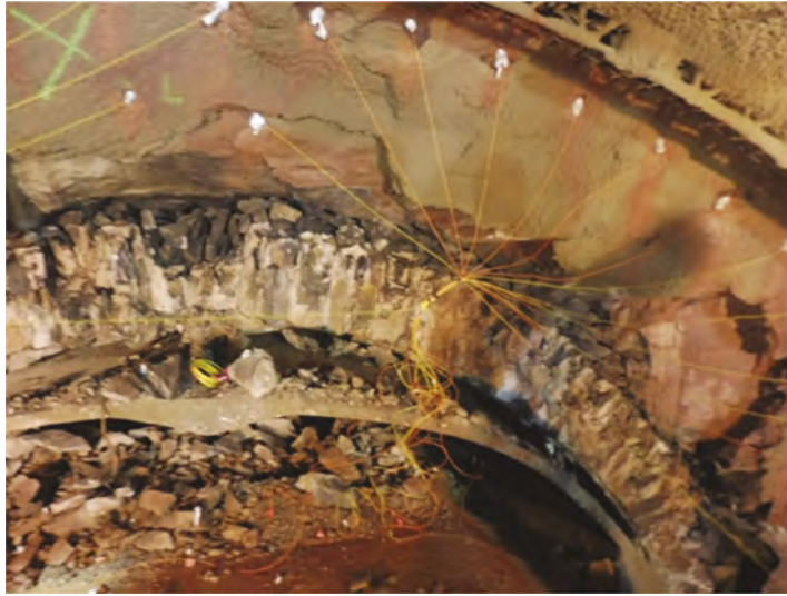
Figure 6. Excavation with drill hammer.
