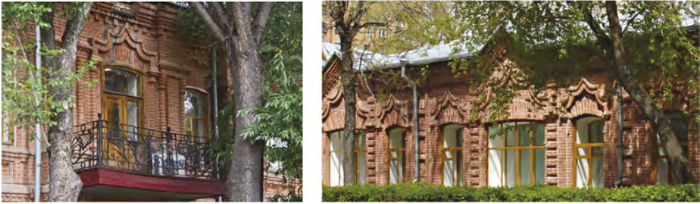
Figure 12. House of the merchant Strelov - was built at the end of the XIX century, 1891.
