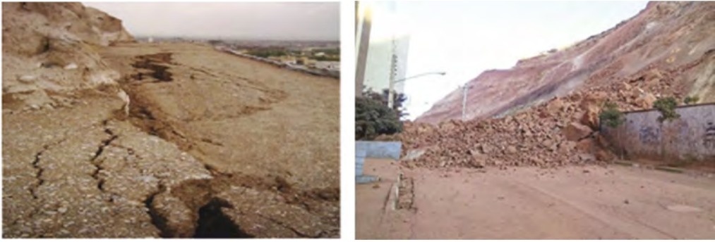
Figure 7. Some pictures of the landslides that occurred in the marl layers in the east of Tabriz.
