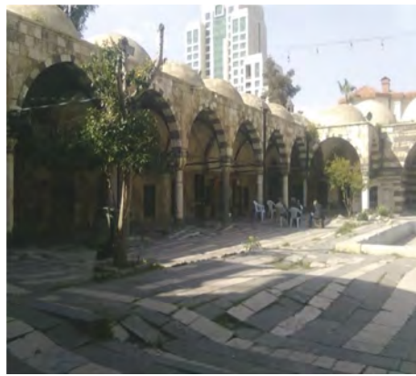
Figure 2. Waves in the soil surface under slabs.
