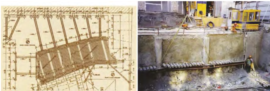
Figure 6. (a) Plan of the temporary support system for the construction of the building. (b) Construction of the fore poles under the antiquities.
