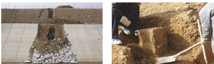
Figure 2. Field sampling of cement modified soil.
