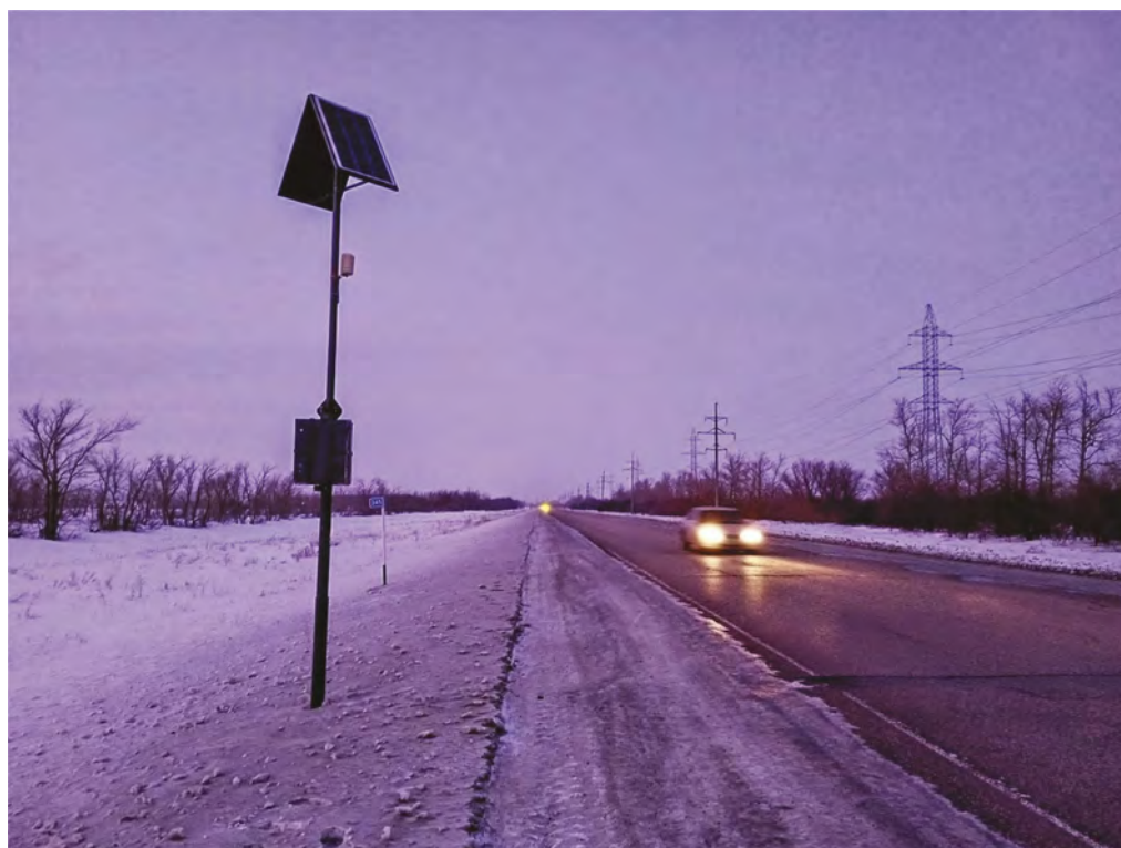
Figure 3. Temperature and humidity monitoring station along the road.
