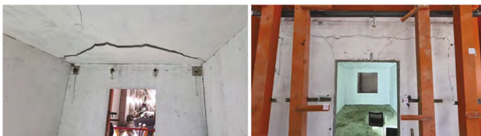
Figure 6. Splitting of the block floor slab No. 2.
