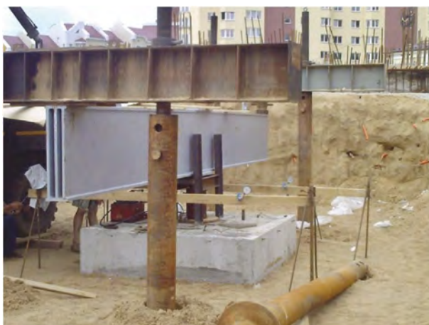
Figure 3. Field static load test.
