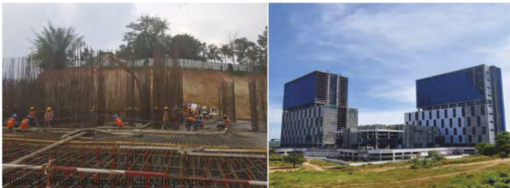
Figure 4. (a). Foundation work in progress (b). Current status of the project.
