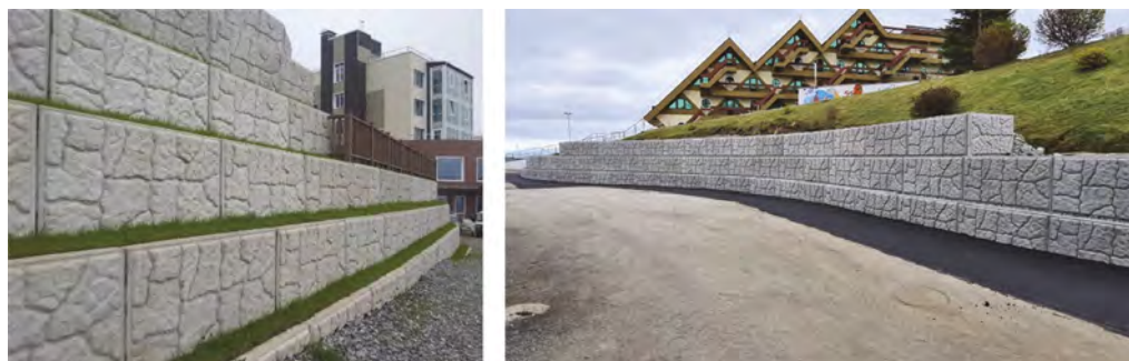
Figure 3. Retaining structures comprised of infilled blocks with greening (Vladivostok, Russia).
