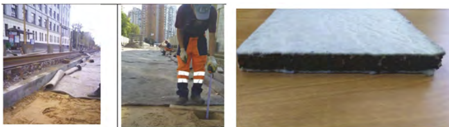
Figure 6. Installation of tram tracks with vibration-proof mats, monitoring.
