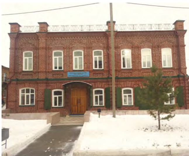
Figure 2. Figured Sandrik above the windows.
