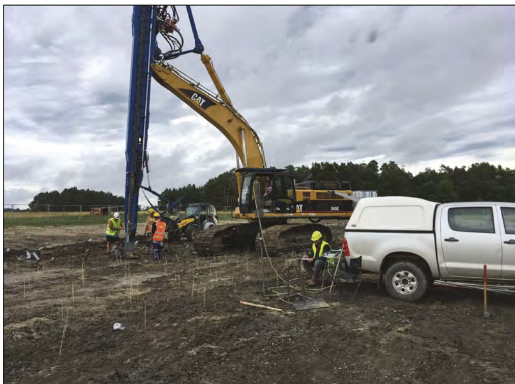
Figure 2. Dynamic penetration probes made during the redevelopment of subsoil with geo-drains.
