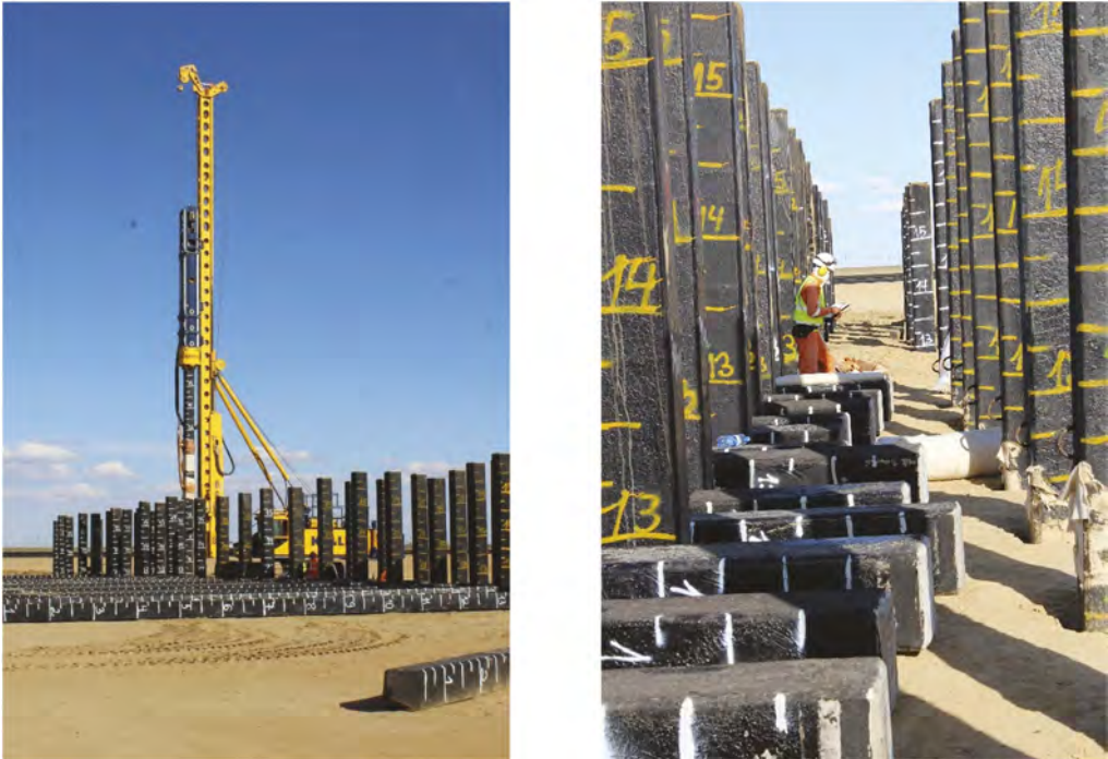
Figure 7. Concrete precast piles at Generator 1, area 52.
