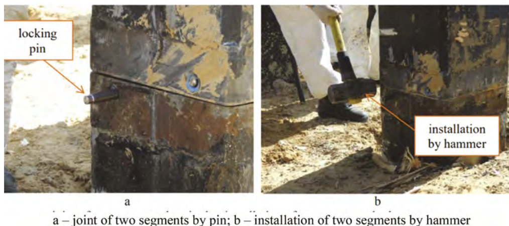
Figure 6. Installation of two segments of PCJP.
