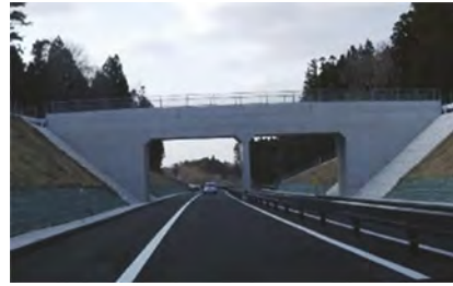
Figure 2. Example of a box culvert type.
