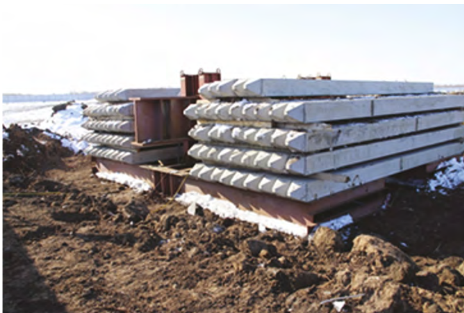
Figure 2. Test piles static loading method SLT by GOST.
