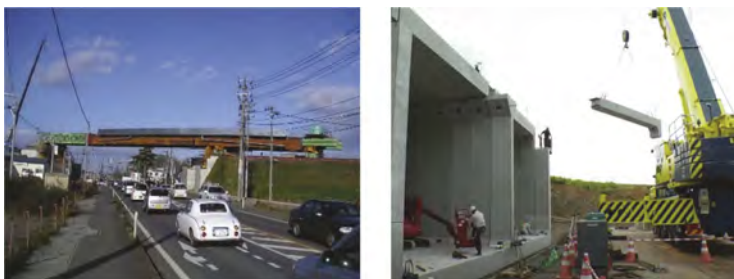
Figure 5. Construction site of girder bridge (left) and box-culvert (right).
