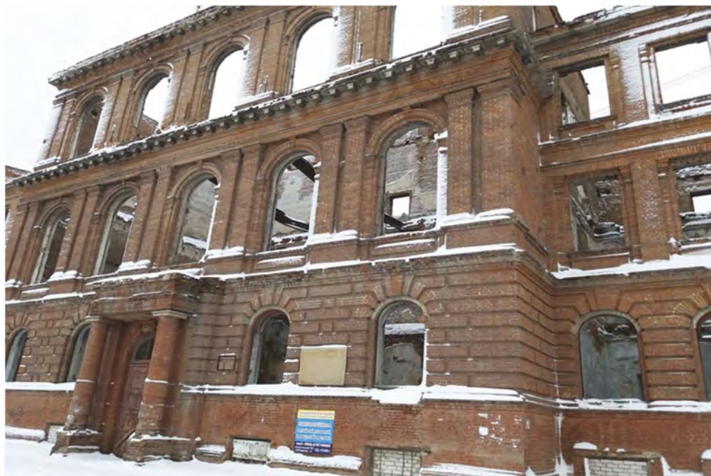
Figure 7. Current view of the former Semey Veterinary Institute building.
