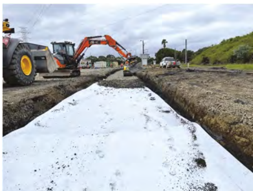
Figure 2. Geocomposite installation to mitigate the fluidization potential of soft soil at Chullora, New South Wales (an ongoing pilot study supported by Sydney Trains).
