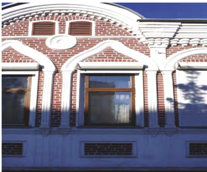
Figure 1. Crowned cornices with ribbon toothed brick brackets.
