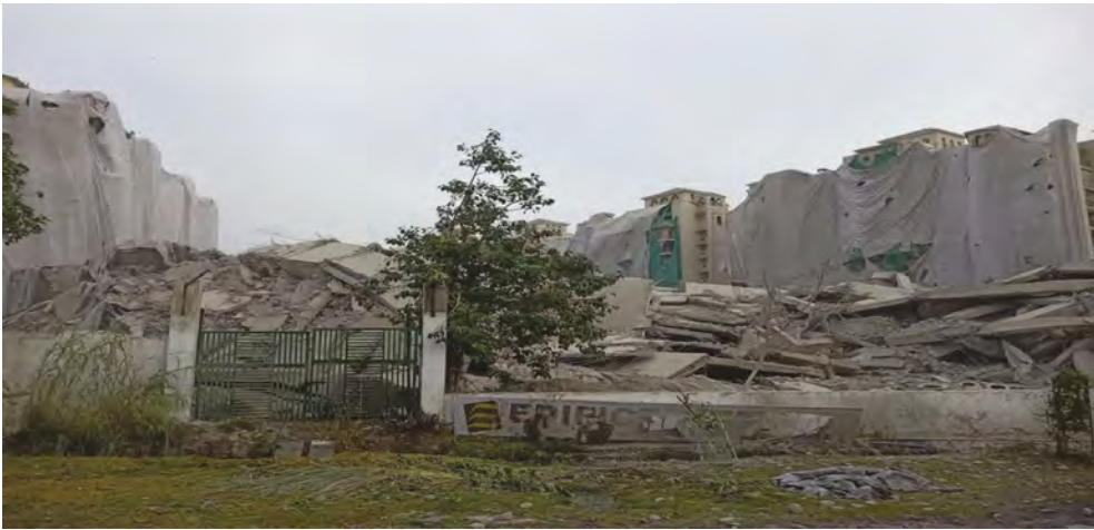
Figure 11. Structure after the collapse.
