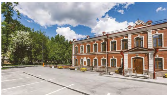
Figure 7. “Tekutievo hospital” after restoration.
