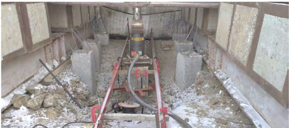
Figure 3. Reference system with displacement transducers, hydraulic jack Enerpac CLS 2006, Load cell Comp load 100t.
