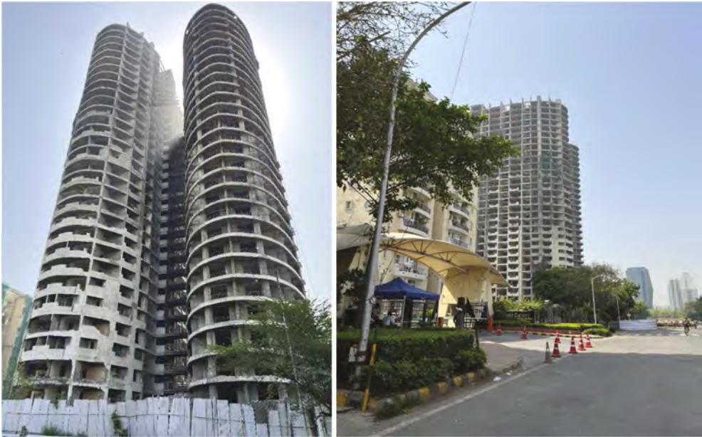
Figure 2. Supertech Twin Tower, Noida before demolition.
