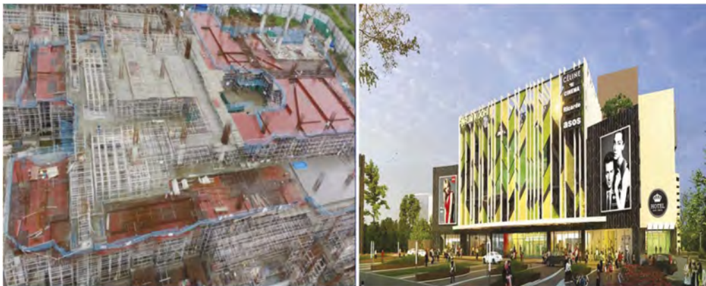
Figure 10. (a) Project during construction (b) Current status of the project.
