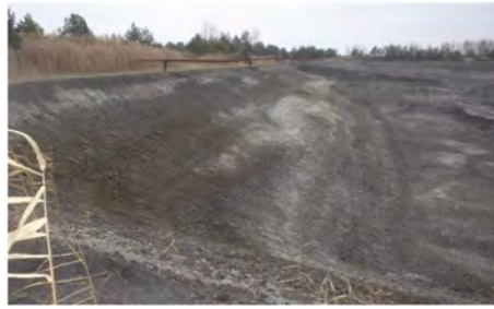
Figure 4. Embankment of the combustion waste landfill “Jelnia” in Stalowa Wola (Poland) constructed from ashes (November 2020).
