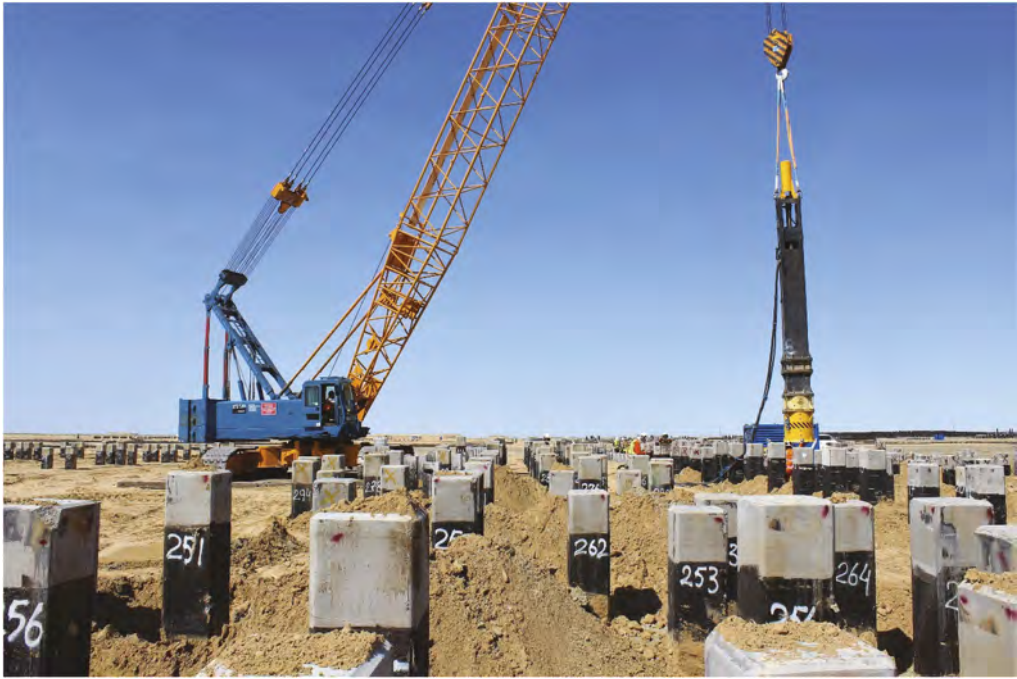
Figure 8. Retapping activity with crane suspended hammer.
