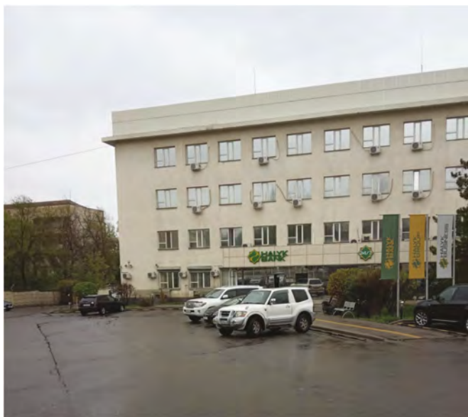
Figure 1. A frame-brick building with installed engineering and seismometric station.
