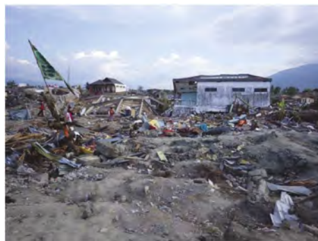
Figure 2. Accumulation of earth and debris at the terminus of Balaroa slope failure.
