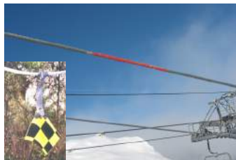
Figure 10: Checkered flags or red paint lines on cables for catex.
