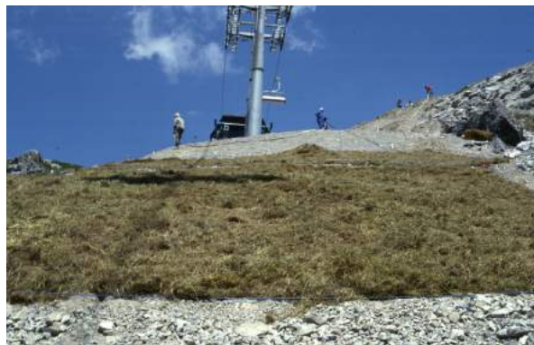
Figure 7: Suitable re-cultivation techniques ensure sufficient protection for the topsoil (Kapall, St. Anton, Austria, 2370 m a.s.l.).
