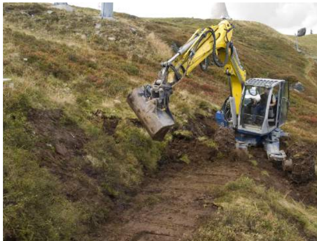
Figure 11: Vegetation turfs collected during levelling are stored for later distribution. They are very suitable for rapidly restoring damaged areas with site-specific vegetation (Hauser Kaibling, Austria, 2000 m a.s.l.).
