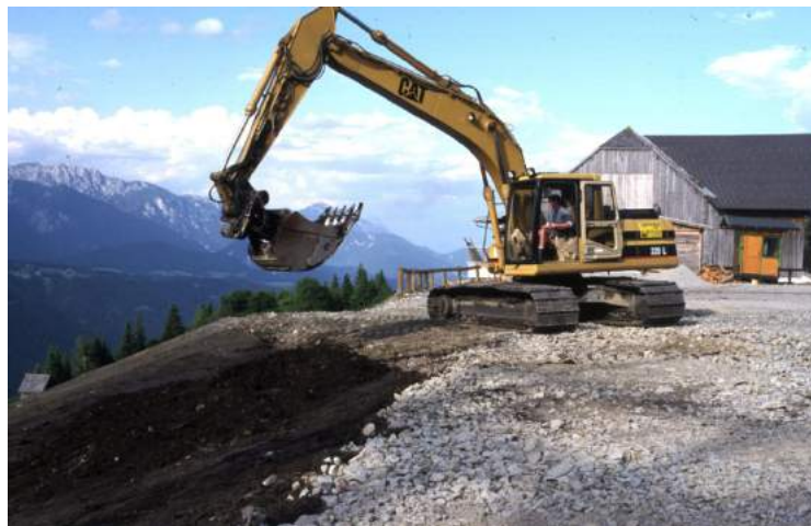
Figure 3: Restoration site at Tauplitz, Austria, 1800 m a.s.l. The available topsoil was carefully collected and redistributed.
