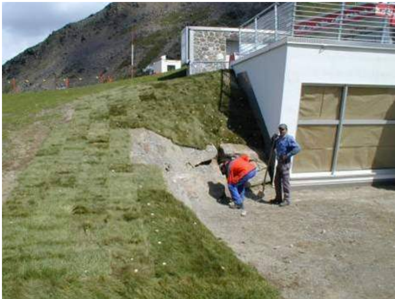
Figure 10: Sod rolls can be used for restorations following small-area disturbances and in extreme locations (Ischgl, Austria, 2400 m).
