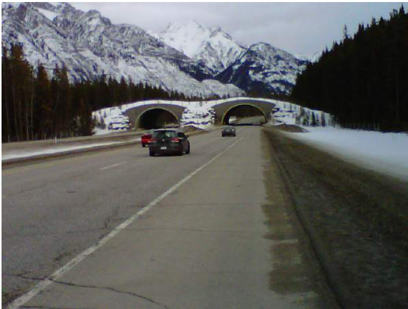
Figure 8: The TransCanada Highway, a railway and the town of Banff are all situated in the narrow valley bottom of the Bow Valley in Alberta. These structures have been found to impede the movements of large ungulates and carnivores. The wildlife connectors shown here have been installed over the highway to reduce mortality and facilitate movements of animals across the valley. Banff-Jasper Highway, Alberta, Canada (Photo by Kathy Martin, March 2011).
