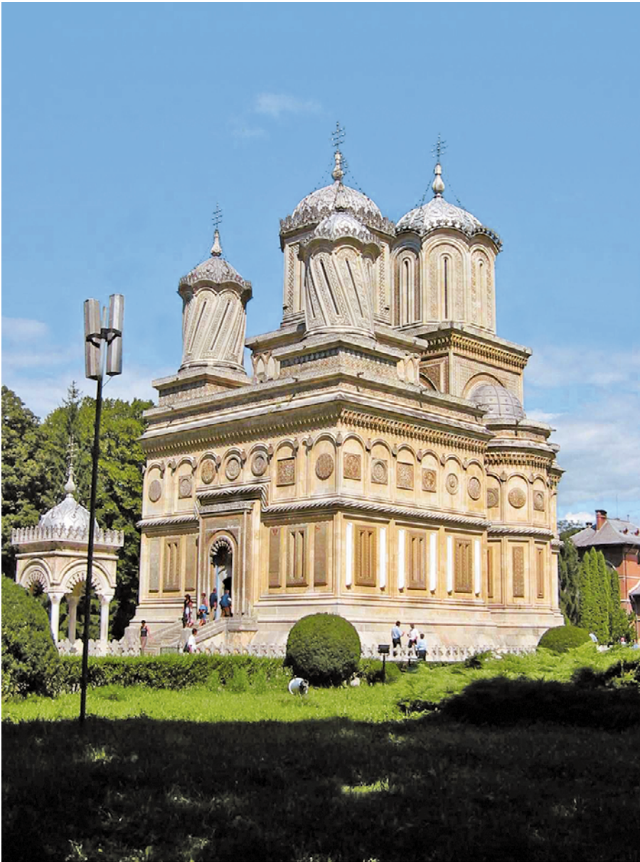
FIGURE 0.5 View of the Royal Monastery of Curtea de Arges, completed 1512–17, Romania PHOTOGRAPH BY THE AUTHOR
