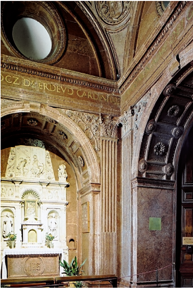
FIGURE 17.1 Giovanni Fiorentino's workshop, Primate Tamás Bakócz's funerary chapel, general view of the altar niche, cathedral, Esztergom/Gran (Hungary), 1507–9. Marmo ammonitico rosso of Tardos (interior), marmo statuario of Carrara (altar) PHOTOGRAPH BY M. WARDZYŃSKI, 2009
