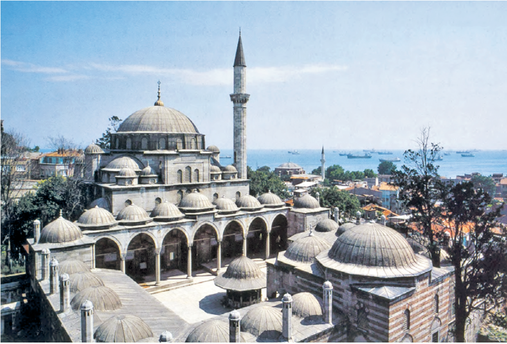
FIGURE 9.3 Mosque complex of İsmihan Sultan and Sokollu Mehmed Pasha, Kadırgalimanı, Istanbul PHOTOGRAPHY BY REHA GÜNAY, FROM GÜLRU NECİPOĞLU, THE AGE OF SİNAN: ARCHITECTURAL CULTURE IN THE OTTOMAN EMPIRE , LONDON, 2005
