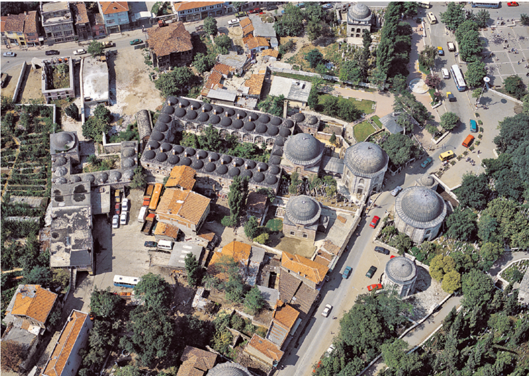
FIGURE 9.4 Funerary Madrasa complex of İsmihan Sultan and Sokollu Mehmed Pasha, Eyüb, Istanbul PHOTOGRAPHY BY REHA GÜNAY, FROM GÜLRU NECİPOĞLU, THE AGE OF SİNAN: ARCHITECTURAL CULTURE IN THE OTTOMAN EMPIRE , LONDON, 2005
