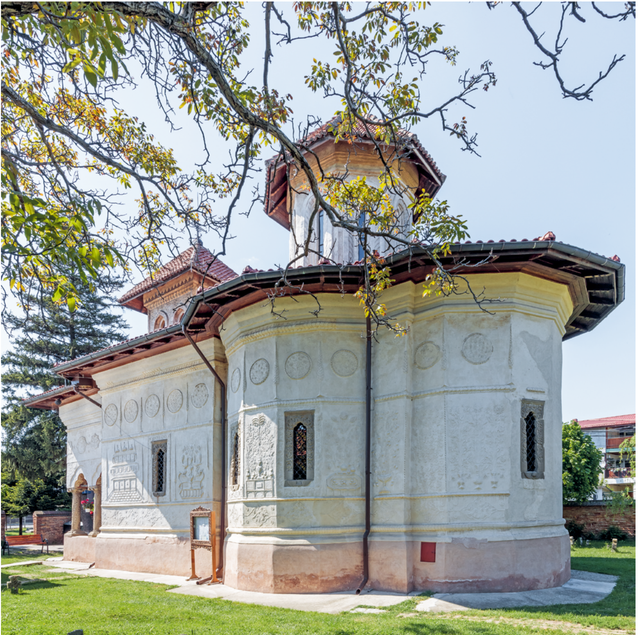
FIGURE 16.6 South-east view, Fundenii Doamnei church, Bucharest PHOTOGRAPH BY SERIOJA BOCSOK, MAY 2021
