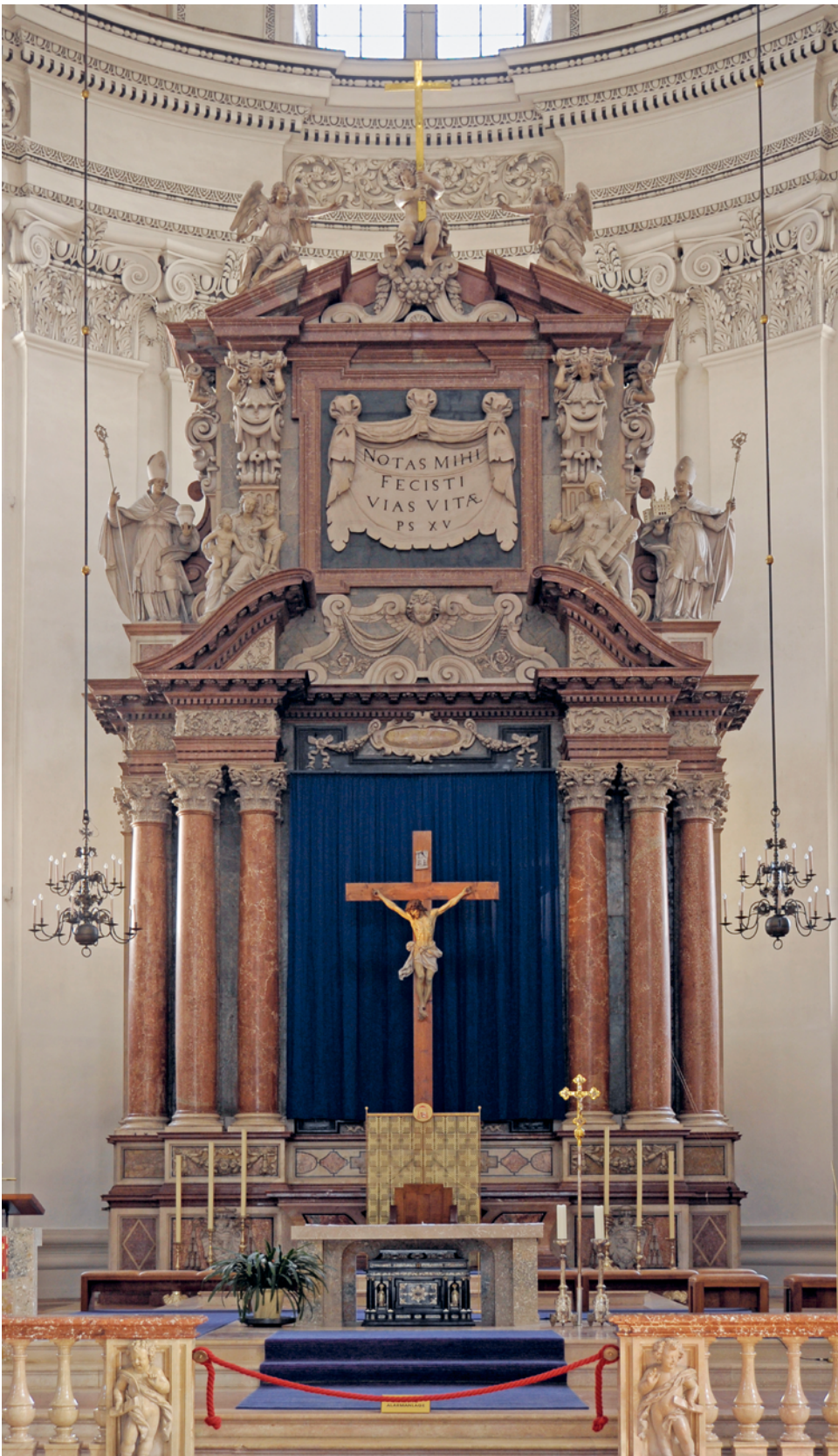
FIGURE 17.4 High altar, Salzburg cathedral, 1628, designed by Santino Solari, executed by Hans Waldburger and Hans Pernegger the Younger of Salzburg. Reddish Jurassic nodular limestones Rot and Rot-grau Scheck of Adnet, whitish limestone Forellenmarmor of Untersberg PHOTOGRAPH BY M. WARDZYŃSKI, 2011
