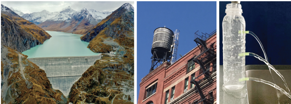
Figure 3.16: Water stacked vertically in vessels. Left: An artificial lake in the Alps (Grand Dixence dam)—water is delivered at high pressure to a hydroelectric power station almost two kilometers below. Center: Water tanks are raised high in order to raise the pressure of water at the tap. Right: Water in a bottle flows with different strengths from different depths.
