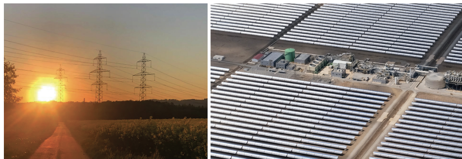
Figure 4.1: Left: From the Sun's light to electricity (photo: PL). Right: Solar thermal power plant (Andasol Solar thermal power station in Andalusia, Spain): parabolic trough mirrors concentrate the Sun's light upon a pipe carrying a synthetic oil which is heated to about 400°C. The heat of the hot oil then powers a thermal power plant; the thermal power plant can be seen at the center of the field. See also Fig.2.8 (left).
