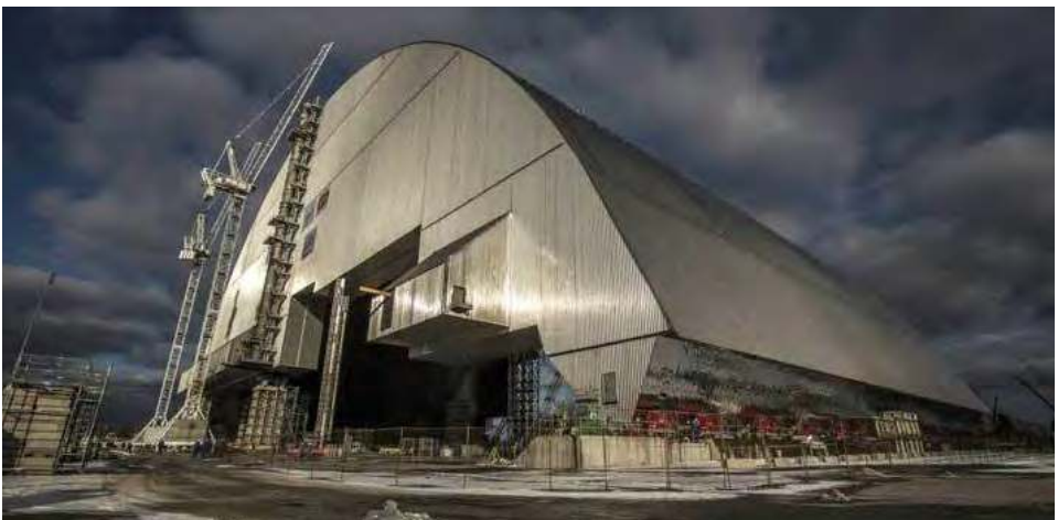
In November 2016 the New Safe Confinement was moved over the old sarcophagus housing the destroyed reactor 4. © EBRD
