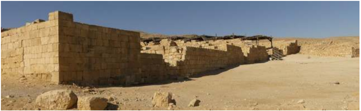
Figure 12. Northern wall of army camp and commander residency (photo O. Sion).
