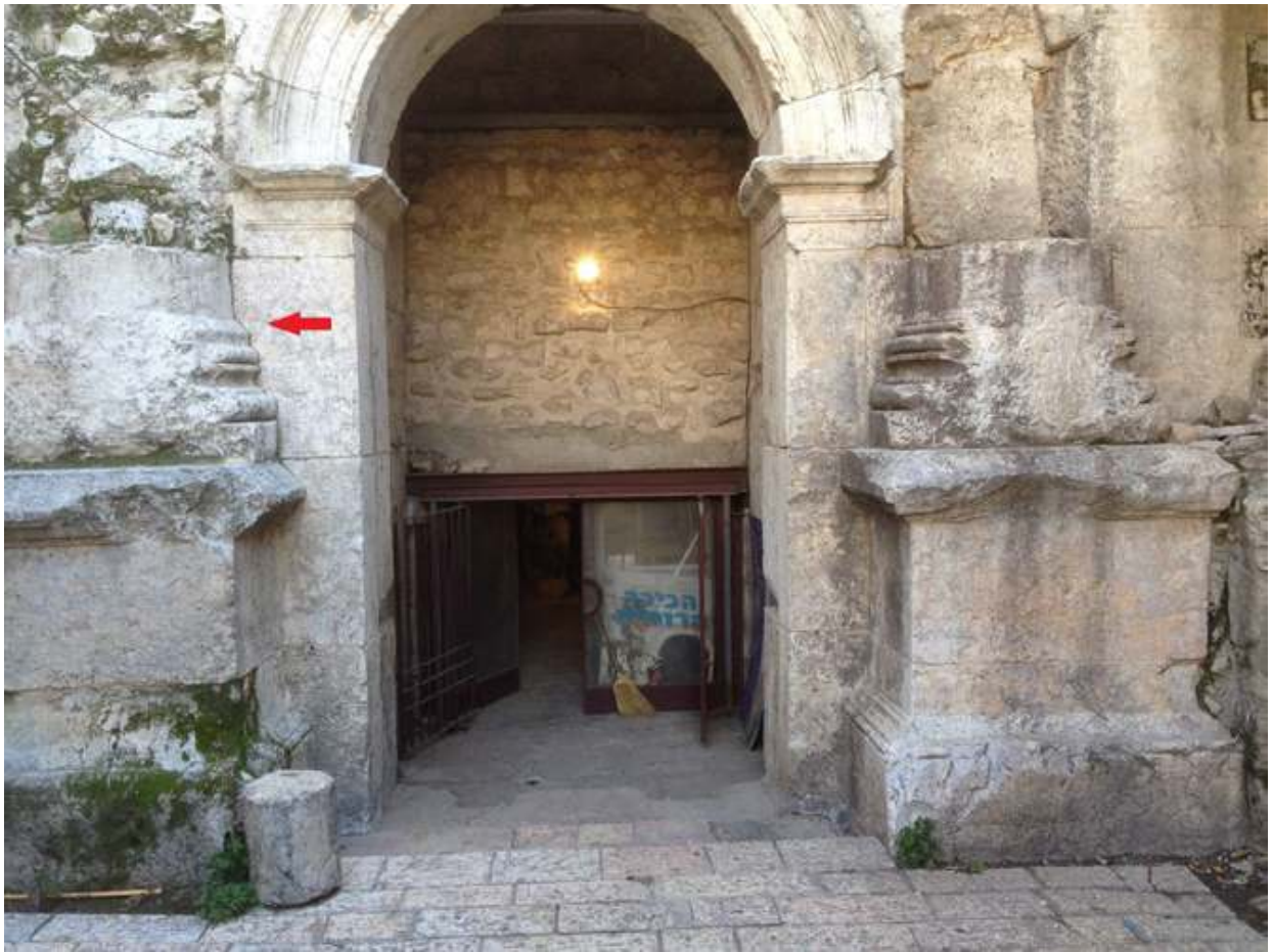
Figure 7. The eastern opening of the Northern Gate of Aelia Capitolina, looking south-east. Pay notice to the blocked-out apophyge on the column base to the east (left) of the opening (Shlomit Weksler-Bdolah).
