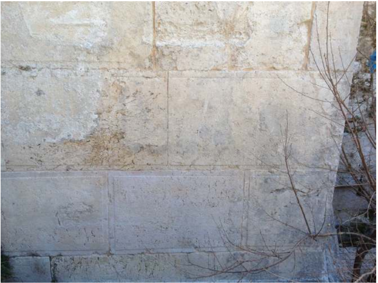
Figure 8. The eastern tower of the Northern Gate of Aelia Capitolina with several ashlars, whose drafted margins are not fully carved. Looking north-east (Shlomit Weksler-Bdolah).
