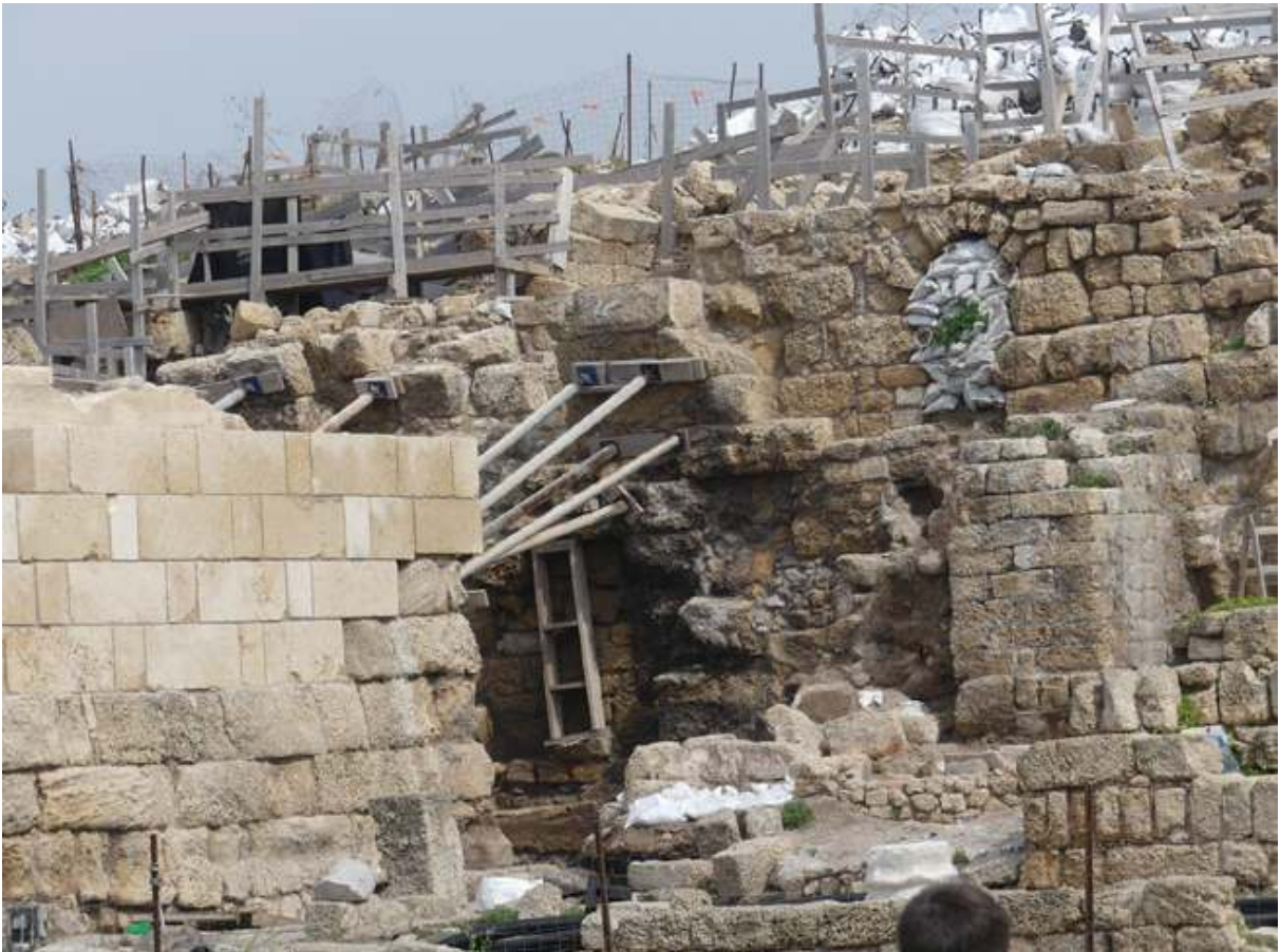
Figure 7. The stones of the eastern arch incorporated in the façade of the small vaults. Note that the height of one of the small vaults rises high above the stones of the arch (Photo: the author).
