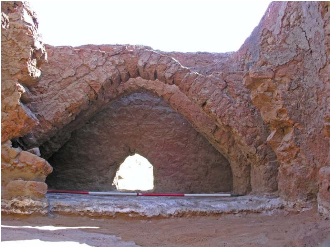
Figure 3. Kawa. The furnace chamber of Building F7 looking towards the eastern stoke-hole. The ash deposits on the floor are visible in section (scale bar 2 m).
