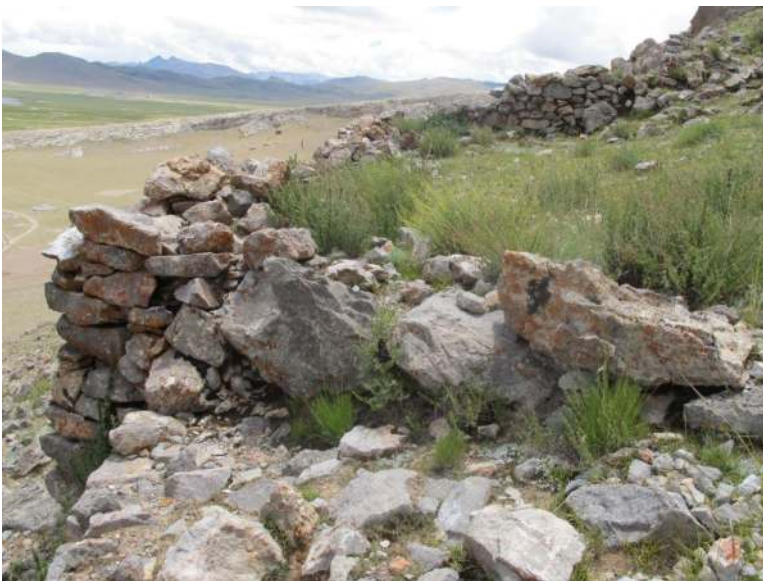
Figure 276. The north (foreground), east wall (left) and south wall (background) of the ostensible edifice at Rdo 'khor phug pa. These walls were built of limestone blocks, some of which appear to have been roughly hewn into shape.
