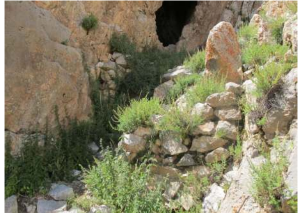
Figure 280. The remains of revetments and a landing just below the mouth of Rdo 'khor phug pa.
