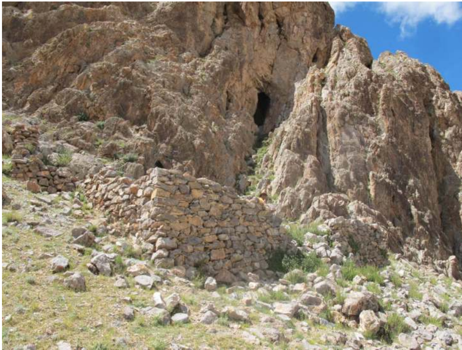
Figure 273. The ruined limestone hulk below Rdo 'khor phug pa as seen from the southeast. This structure is underpinned by a prominent revetment. Note the extension of the south wall (far left) well beyond the bounds of the building.
