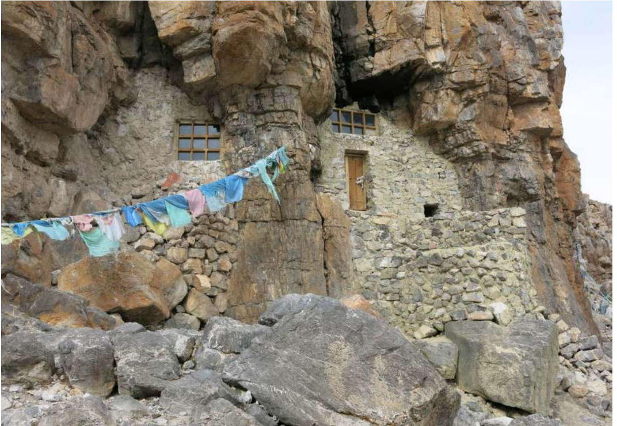
Figure 218. Glang chen phug, Gyer ru mtsho do. As can be seen in the image, the cave is divided into two parts. The right half functioned as a kitchen and fuel storage area and the left (with large window) was used for religious practice and sleeping. The latrine is placed below the kitchen.
