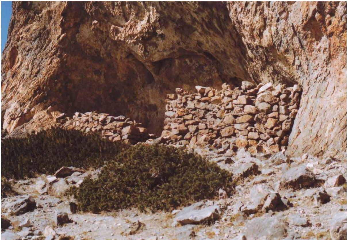
Figure 139. S3_L7 with its massive front wall, which is 11 m long, 70 cm thick, and as much as 1.5 m in height. Inside this wall there are two internal partitions now reduced to 1.7 m and 2 m in length.
