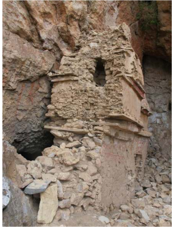
Figure 310. The twin chortens act as a front structure to the recess on the west side of the overhang. A portion of the fire-blackened roof of this sheltered space can be seen at the bottom left side of the image. Note the use of large stone slabs between each main stage of the chorten .
