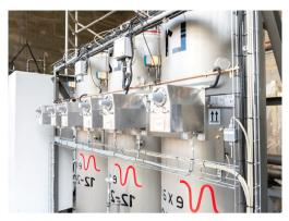
Figure 9.1.4: 10 kV, 40 MVA resistive type superconducting fault current limiter [Schmidt2015]
