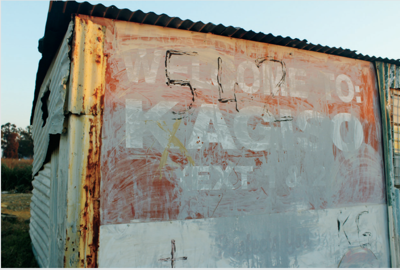
4.13 A faint yellow X on the wall of a shack built in part from an old sign welcoming people to Kagiso Extensions 1 and 2. Mr. Ramoruti asked me to take this photo to prove that nothing had changed in the four years since the shacks had been marked. G. Hecht.
