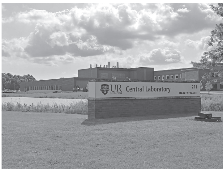
Figure 38. University of Rochester Central Laboratories at Bailey Road (2019)
