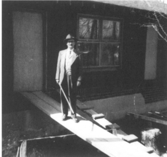
Figure 16. Walking the plank in front of his new house, 1954. Lee Reynolds contracted and built the new home according to Cratis’s and Libby’s design. The house was the first one on what for many years was called Reynolds Road.
