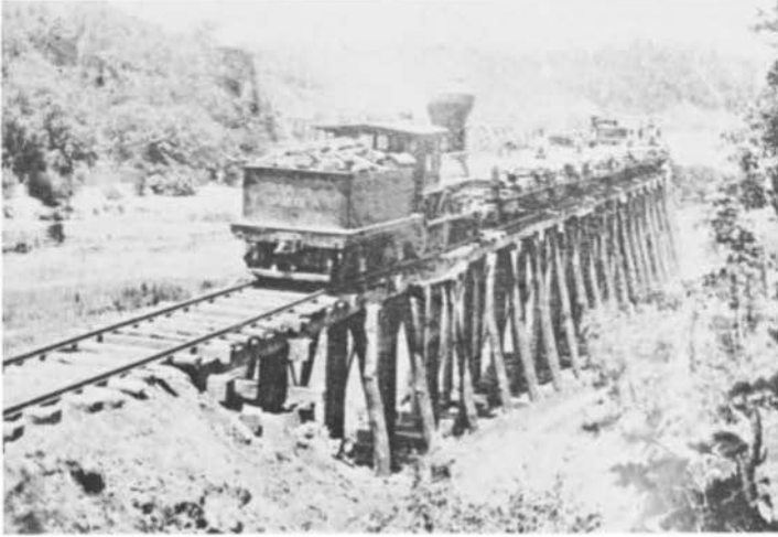
Hauling wood to build the Western North Carolina Railroad. The engine at the front is the little Salisbury that was hauled over the mountain to expedite the digging of the Swannanoa tunnel ASHEVILLE CITIZEN-TIMES CO.
