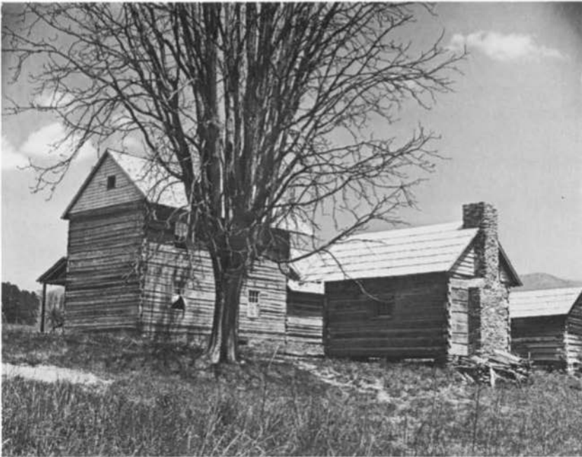
Vance Birthplace after restoration
