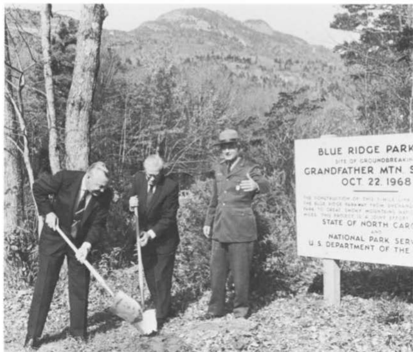
Ground breaking for final link of Blue Ridge Parkway by Governor Dan Moore and Assistant-Director of the National Park Service
