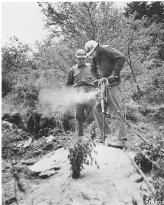
CCC men learned to use power tools.
