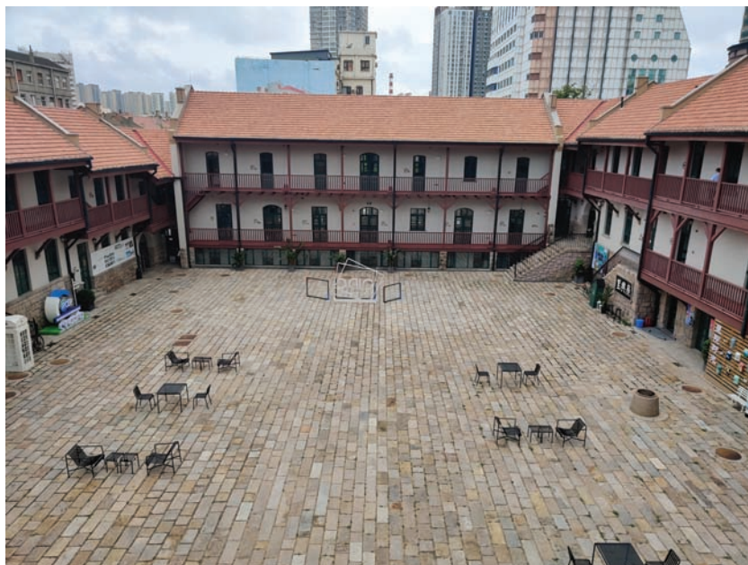
Fig. 11. Guangxing li after refurbishment (fieldwork photo, 2021)
