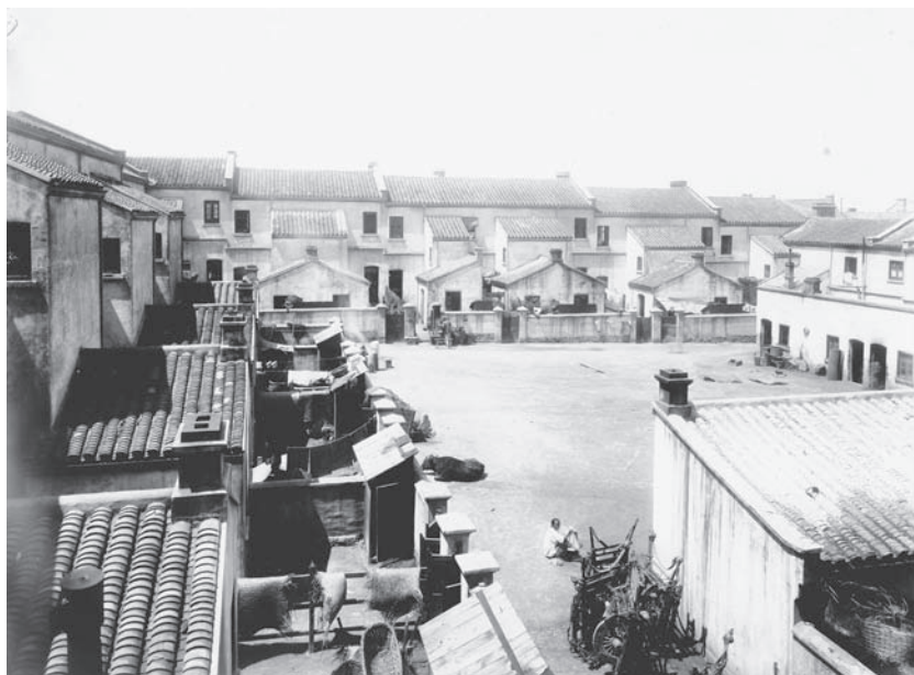
Fig. 1. One of the first courtyards built by Alfred Siemssen in Qingdao (courtesy of the Siemssen family)
