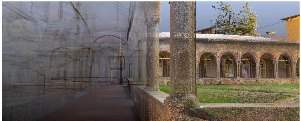
The main cloister of the former convent of San Francesco: restitution of the integrated model.
