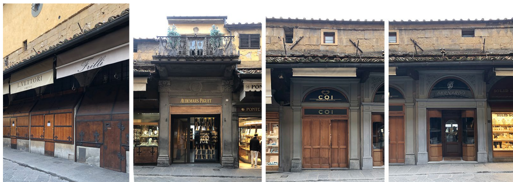
Fig. 3. From left, characteristic commercial front of Ponte Vecchio with the 'madielle' display system. Shop front of the former Luigi Ricci goldsmith's shop at 16/r, restructured to a design by Martelli in 1857. Two characteristic shops restructured during the 19th century as variations of Martelli's design. Photograph by the authors.
