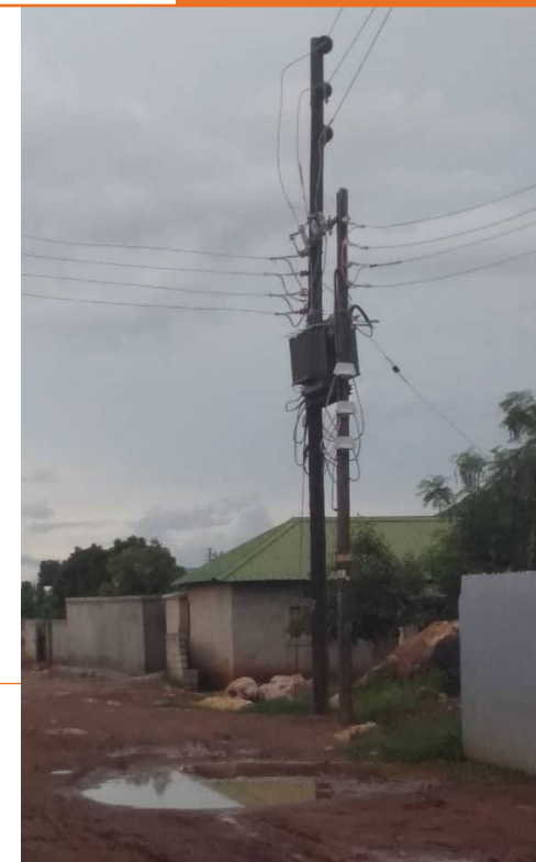
Electricity Transformer and Grid distributed above ground cables at low voltage within the City of Lusaka, Zambia.
