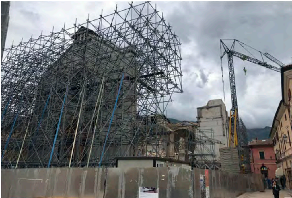
Figure 12. The metal scaffolding framework of the Basilica of San Benedetto.
