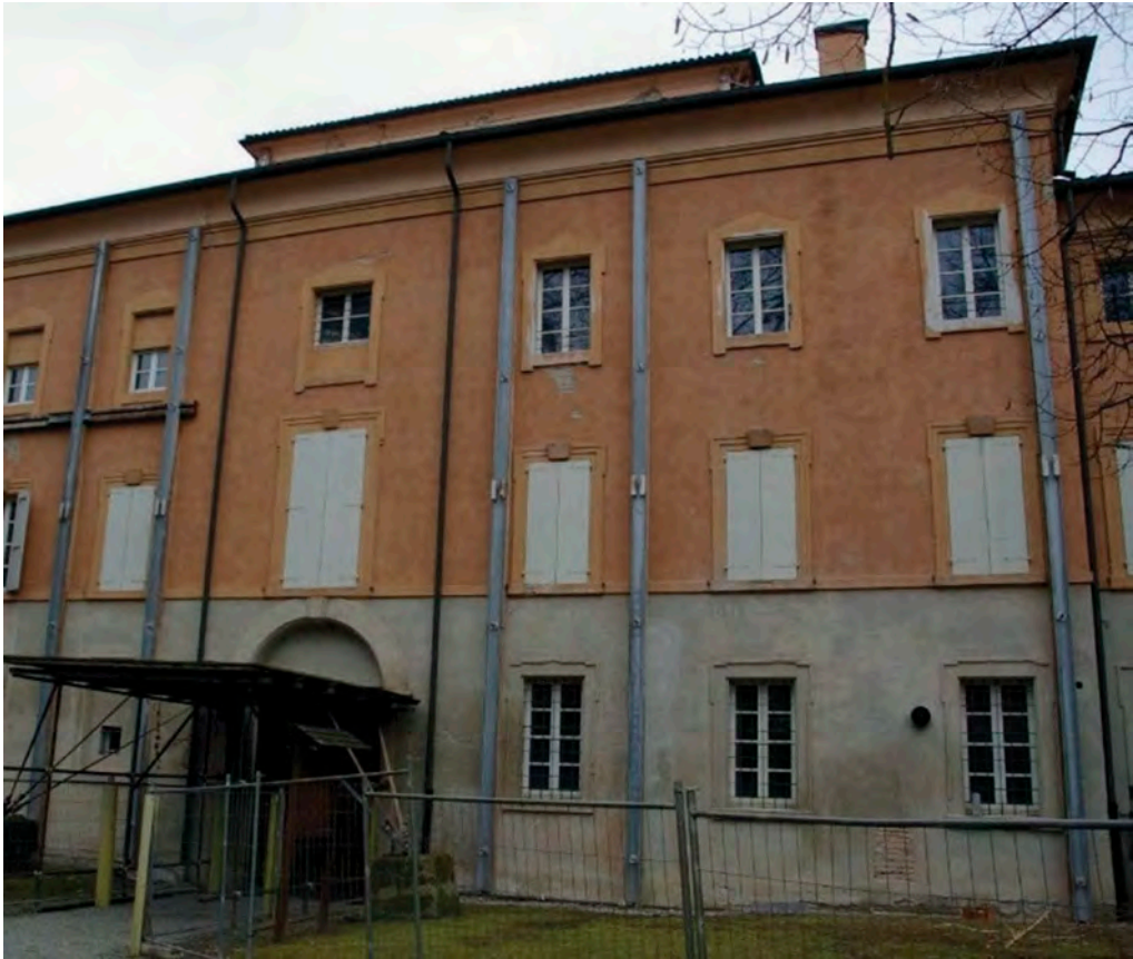
Figure 7. The back of Palazzo Sartoretti opening onto the large park. The works to make it safe included large steel pillars and chains to prevent the brick walls from collapsing out of level.
