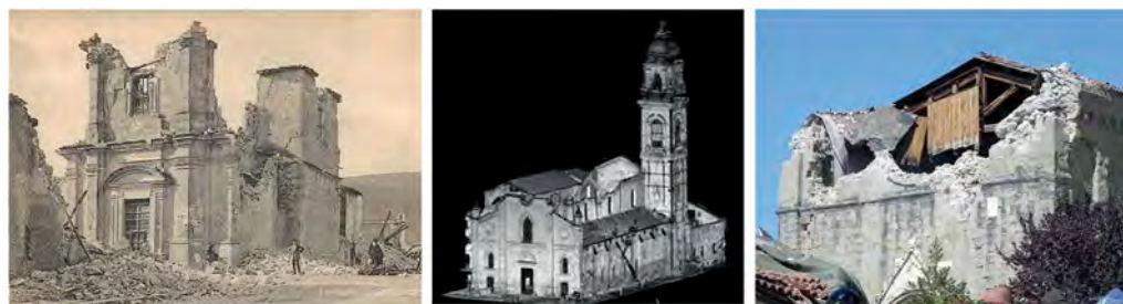
Figure 1. The overturning of the faade is one of the most recurring damage mechanisms in masonry churches: here just some examples taken from different Italian earthquakes in the last century: from left to right, 1915 San Giovanni Church in Avezzano (AQ), 2012 Santa Maria Maggiore Church in Mirandola (MO), 2016 Church in Amatrice (RI).
