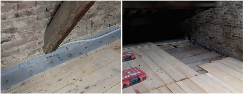
Figure 15. Stiffening of attic slabs and metal curbs.
