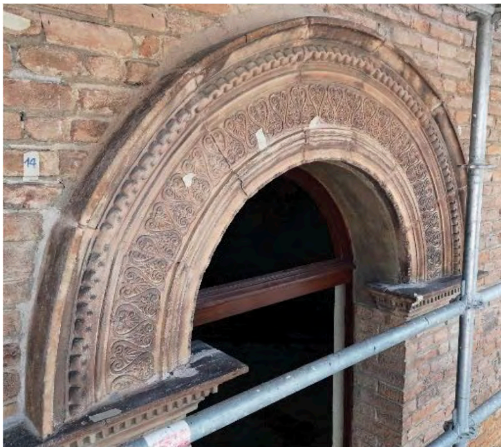
Figure 22. Restoration of plaster fragments and window surrounds.
