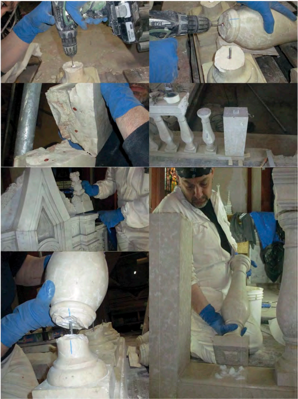
Figure 31. The Altar of the Most Holy Sacrament, assembly process of the stone fragments of the balustrade by gluing, pivoting and cast reconstruction of the missing cusp to the right of the Tabernacle.
