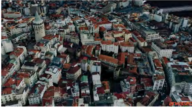
Figure 7. Location of the Genoese defense walls in İstanbul. The remaining walls are connected to Galata Tower on the left and reaches down to Bankalar Street.
