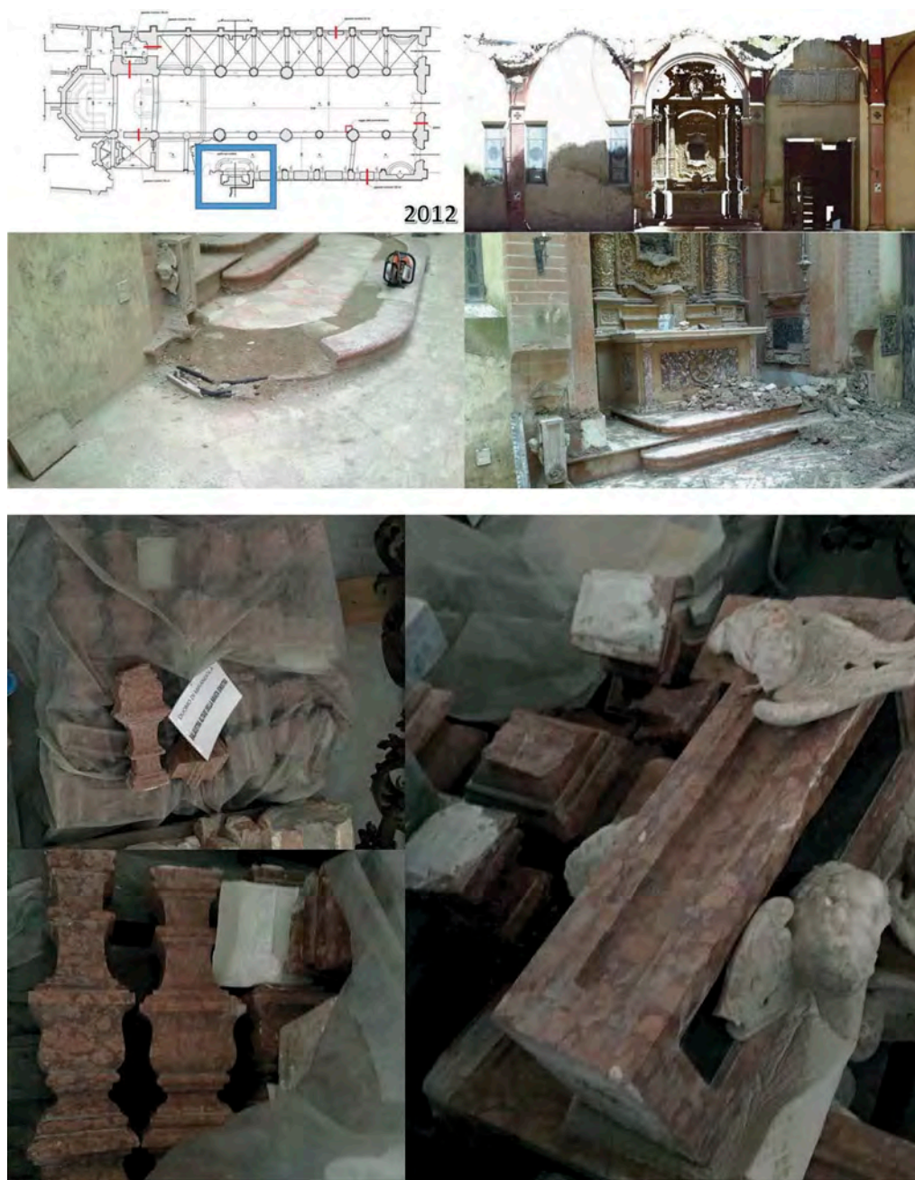
Figures 26-27. The altar of the Rosary, involved in the collapse of the vaults above, suffered extensive damage to the stone balustrade and the two statues located within the side niches. Above, the post-earthquake state of the altar. Below, the benches with all the recovered fragments including the winged putti and their fragmented parts.
