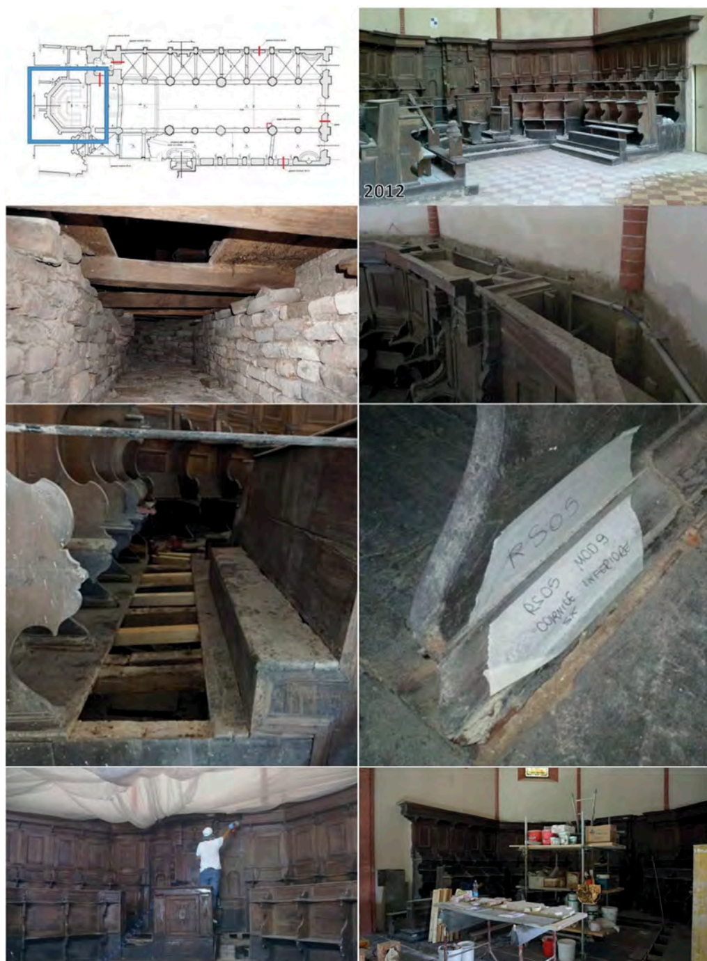
Figure 35. The wooden choir: disinfection, cleaning, repair and shellac treatment.
