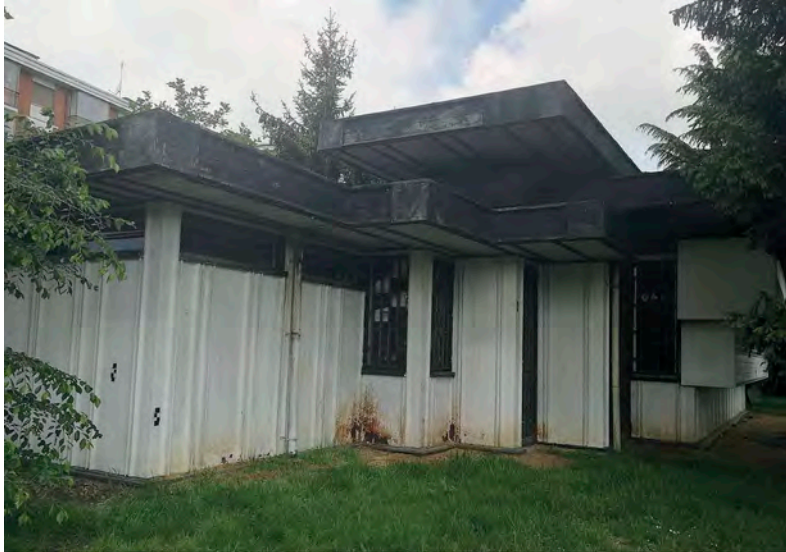
Figure 3. Picture of the actual State of the Library.
