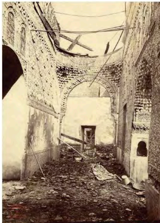
Figure 5. View of barca room after the fire on september 1890.
