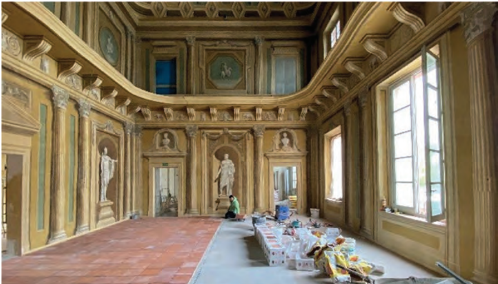
Figure 30. Picture of the Salone during the laying of the terracotta floor after the scaffolding had been removed.
