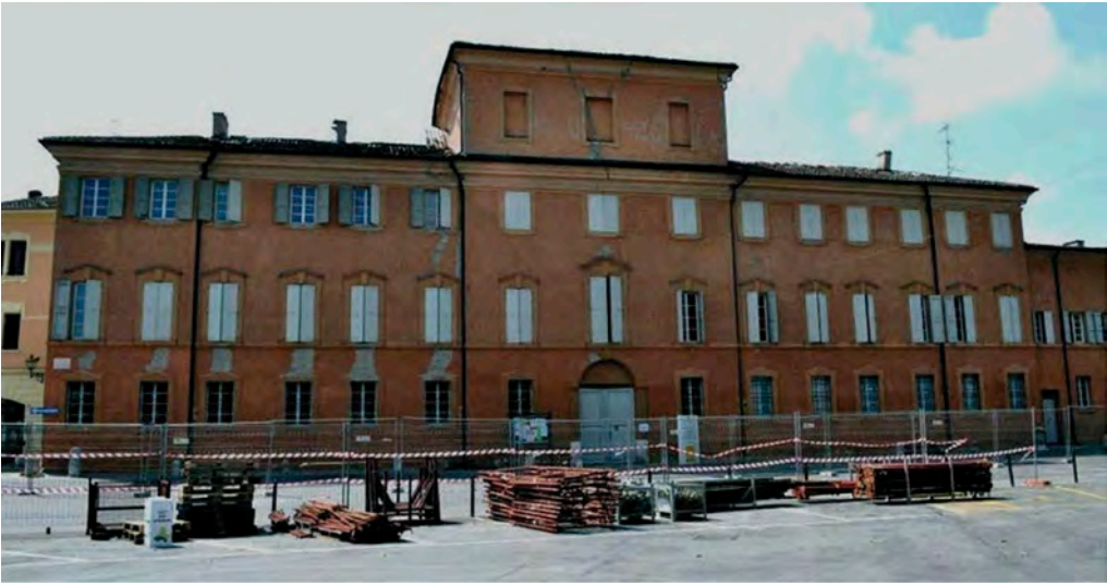
Figure 5. The main front of Palazzo Sartoretti, the backdrop of Piazza Martiri, as it looked after the 2012 earthquake.
