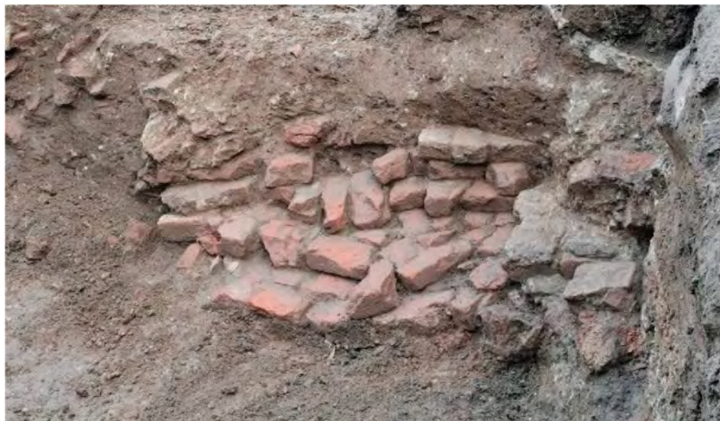
Figure 26. Detail of the foundations of the original external staircase for access to the Salone dei Mesi.
