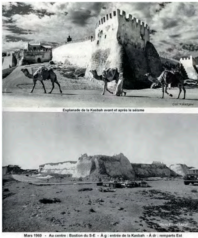
Figure 11. The Walls of the Kasbah, before and after the earthquake.
