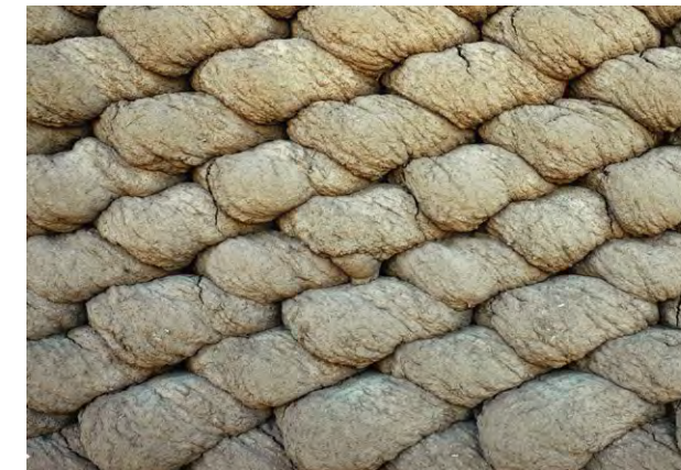
11. Wall texture detail of the 3D-printed adobe surface. © Barrak Darweesh, Ronald Rael, University of California, Berkeley.
