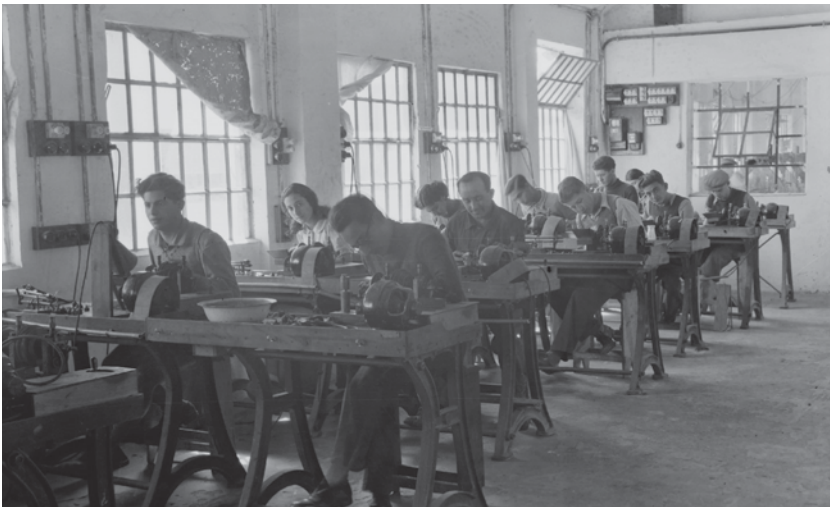
Figure 1.2. Diamond cutting on lathes in Jewish factories in Palestine on Plain of Sharon and along the coast to Haifa. (Tel Aviv. Diamond works, March 1939. Public Domain image Courtesy of the Library of Congress.)
