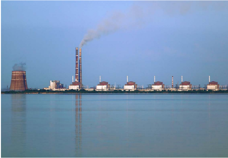
Figure 8.1. Zaporizhzhia NPP viewed from across the Kakhovka Reservoir. The large building between the cooling towers and the reactors, and the two tall smokestacks, belong to the Zaporizhzhia thermal power station, located about 3 km beyond the nuclear plant.
