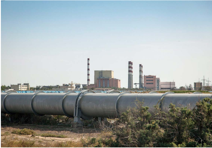
Figure 6.1. Water conduit at Aqtau (formerly Shevchenko), Kazakhstan, leading from the nuclear desalination plant into the city. The reactor building is located between the chimneys.
