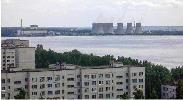
Figure 5.1. View from Novovoronezh showing the cooling pond and in the background the nuclear power plant, as of 2007. The fifth reactor, for which the pond was built, is visible to the upper left, whereas the first four, smaller reactors are hidden behind the cooling towers that supplement the Don as a cooling source.
