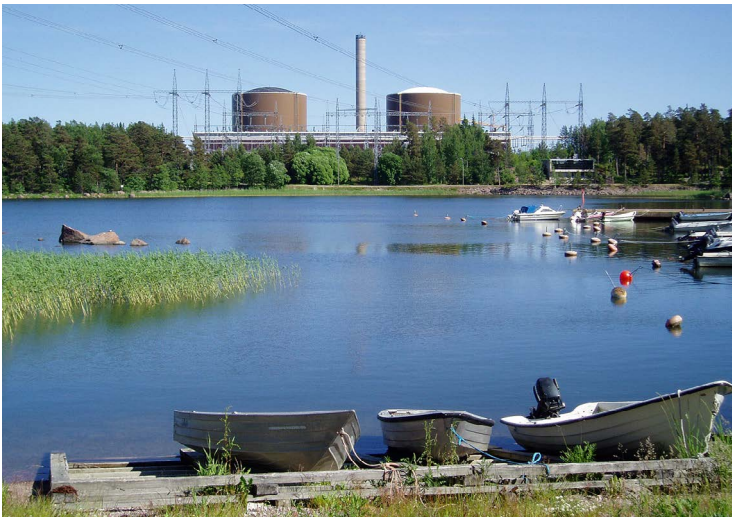
Figure 7.1. Loviisa NPP, Finland. The plant, beautifully situated in the Finnish archipelago, combines Soviet VVER-440 reactors with Western safety components, most visible here through the US-style containment domes. These make the Loviisa plant visually different from all other VVER-440 plants.
