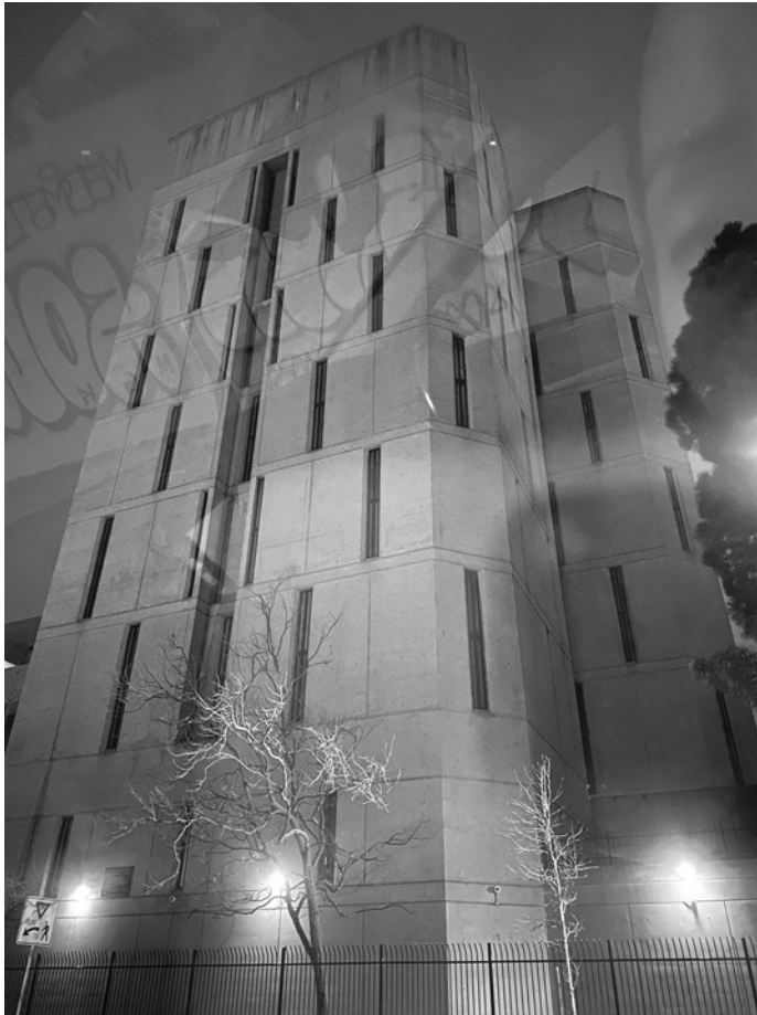
5.9 North County Jail, Oakland, California, 2020. Photo by author.
