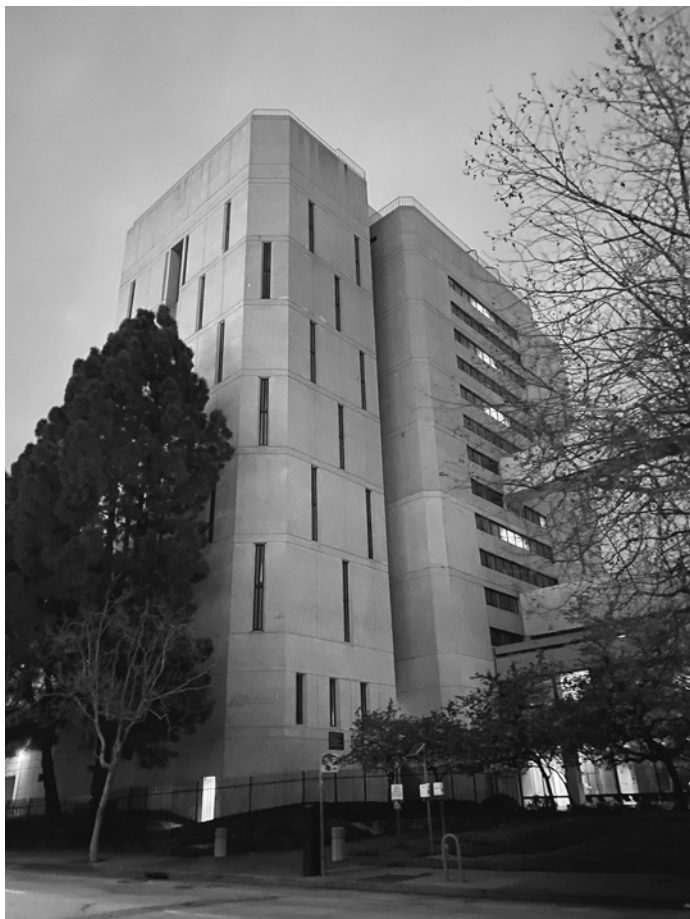
5.11 North County Jail, Oakland, California, 2020. Photo by author.
