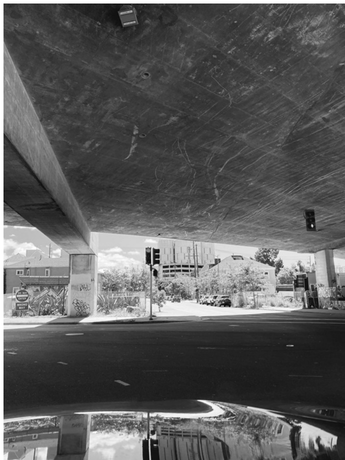
5.4 North County Jail, Oakland, California, 2020. Photo by author.
