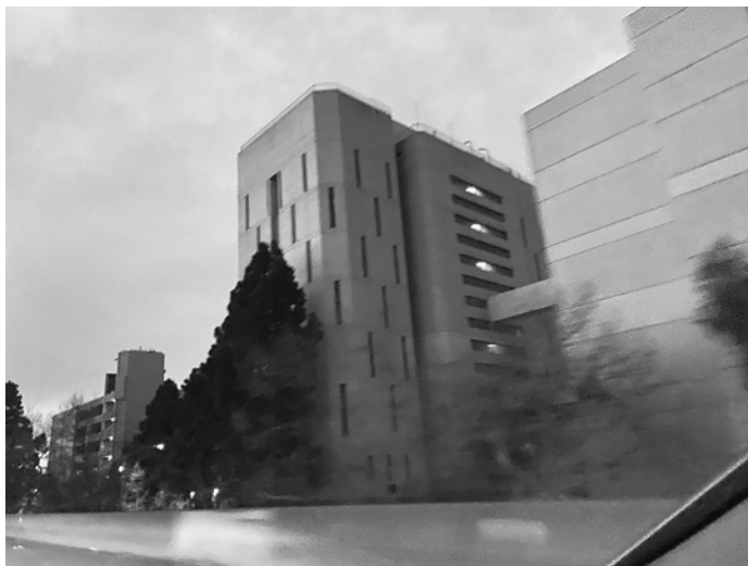
5.1 North County Jail, Oakland, California, 2020. Photo by author.
