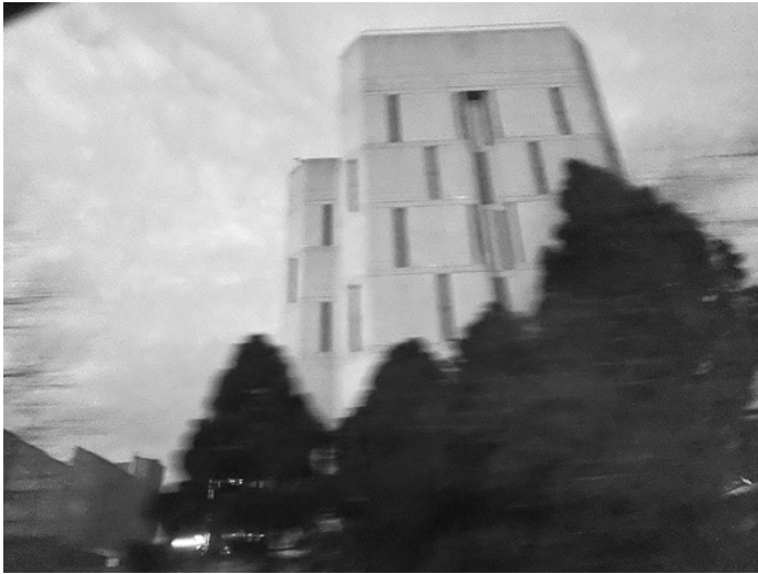
5.2 North County Jail, Oakland, California, 2020. Photo by author.
