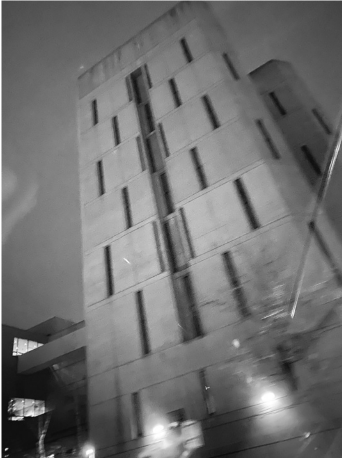
5.5 North County Jail, Oakland, California, 2020. Photo by author.
