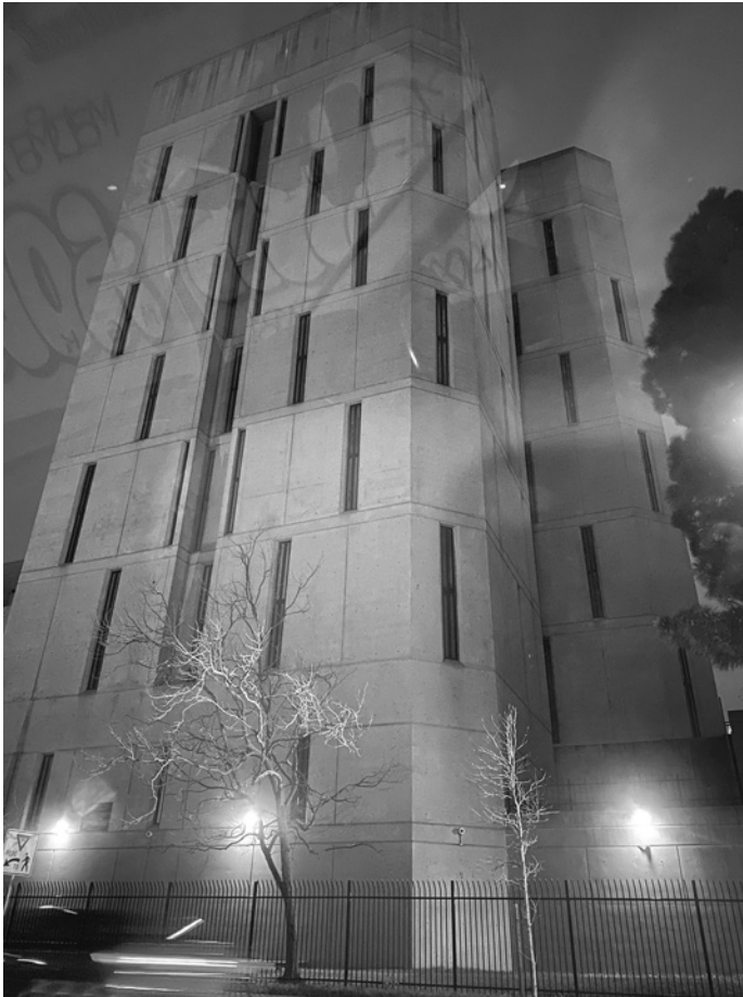
5.8 North County Jail, Oakland, California, 2020. Photo by author.
