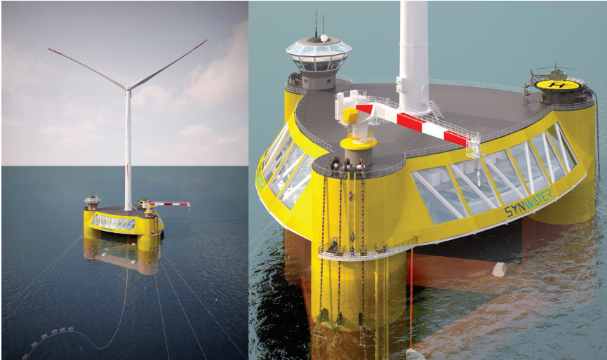
FIGURE 18.3 Floating WINDdesal plant with a capacity of 30,000 m 3 /d for the production of desalinated water (left side: full view including the wind turbine, right side: close-up of the platform) (Synlift n.d.).
