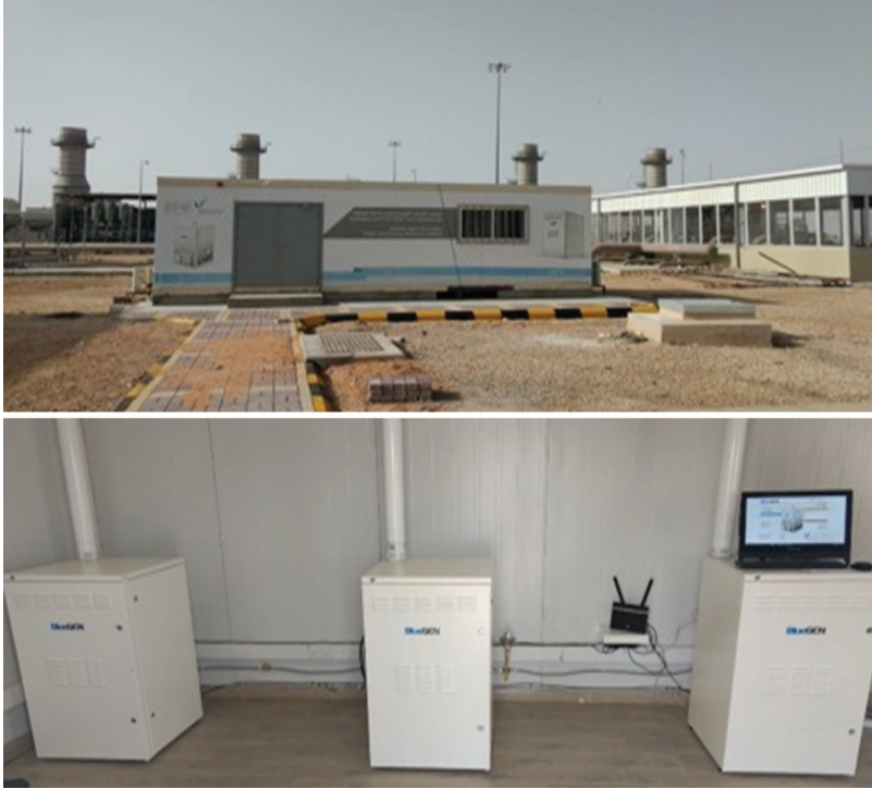
FIGURE 24.10 SOFC system testing facility at the SEC's Power Plant No. 9 in Riyadh.
