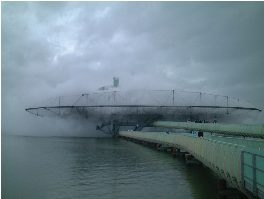
FIGURE 6.1 Diller Scofidio & Renfro, Blur Building , Swiss Expo 2002. Yverdon-les-Bains, Switzerland. Photo: Norbert Aepli. Shared through the Creative Commons Attribution 2.5 Generic license, © Norbert Aepli.
