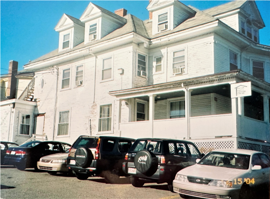
FIGURE 2. Haitian Multi-Service Center, main building, ca. 2004. Photo credit: Robert L. Powell.
