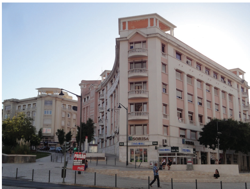
FIGURE 3.2 Even though the expansion of the Avenida da Liberdade boulevard was only partially realized, the neighborhoods created as part of the project are among the most popular residential areas in Lisbon.
