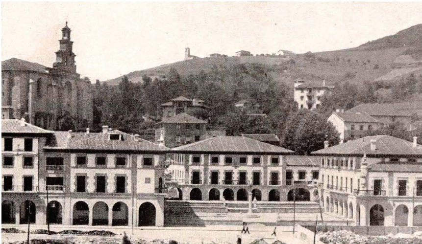
FIGURE 2.5 The civic centre of Franco’s Gernika bears the hallmarks of an applied programme of Spanishness, with a main square set against the commanding backdrop of the church. The award of the work to a renowned Basque architect and the use of local raw materials inspired acceptance among the region’s population.
