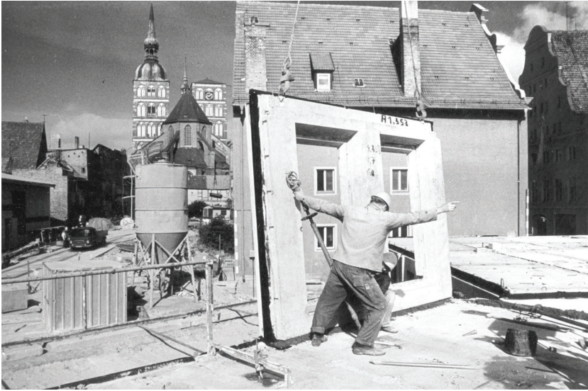
FIGURE 9.5 Planning in small steps: A worker places a slab in a construction area of Stralsund’s old town with just 100 residential units. Photo: Harry Hardenberg, source: Municipal Archive Stralsund, VIII-17-03-115.
