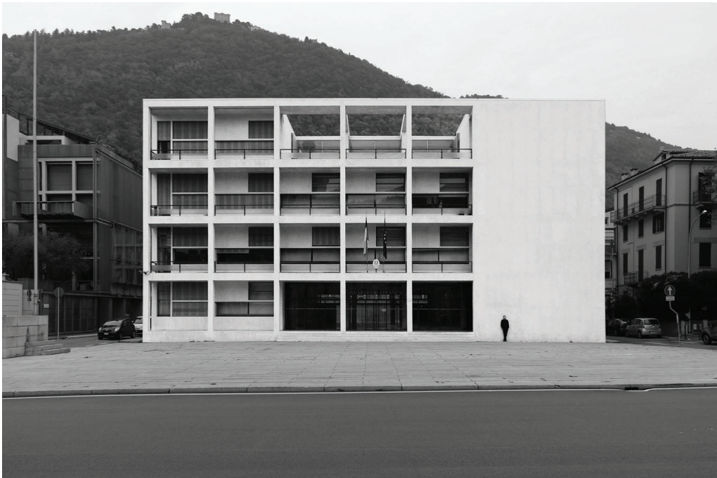
FIGURE 6.1 Como, Casa del Fascio, Giuseppe Terragni, 1932–1936. Photograph by Danny Alexander Lettkemann, 2017.
