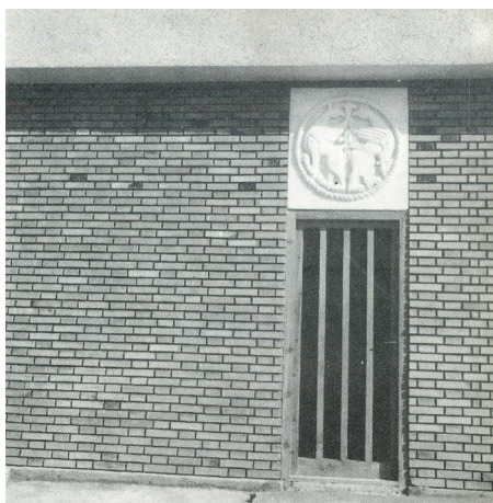
Figure 7-2–Figure 7-6 Gevgelija customhouse, Mihajlo Mitrović, 1965, details. Source: Mihajlo Mitrović, "Zapis o tri moja dela," 1970.
