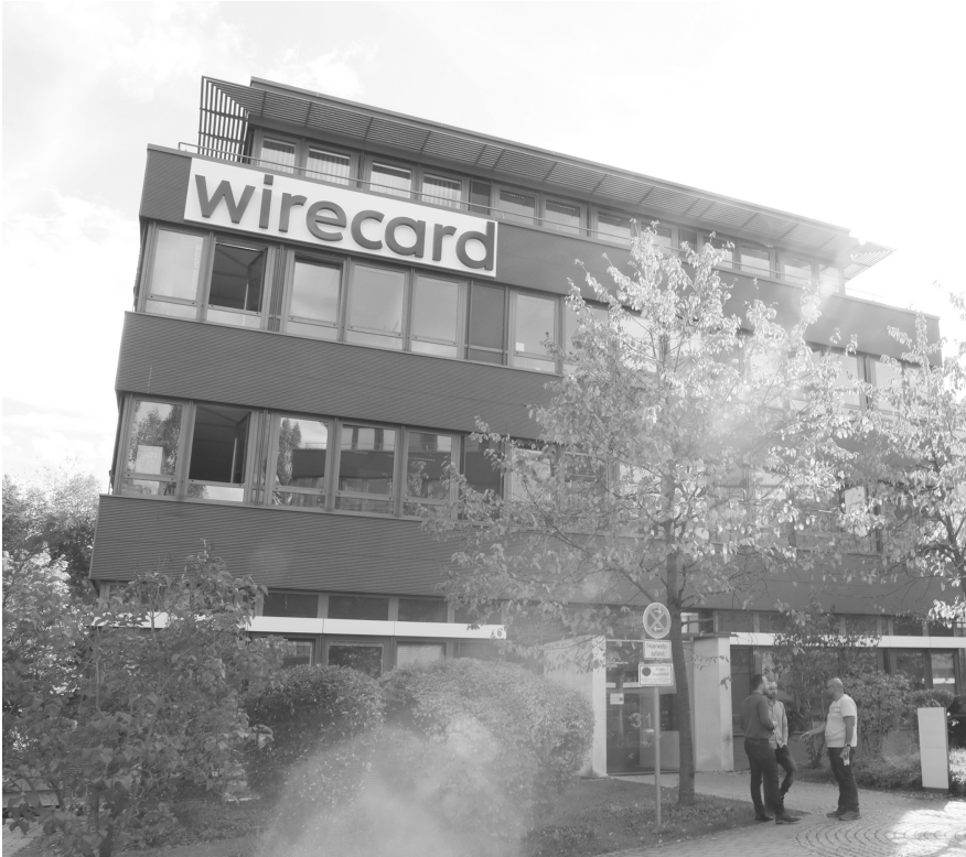
Fig. 2: Wirecard Headquarters, Aschheim. Photo: Leo Molatore, CC BY-SA 2.0.
