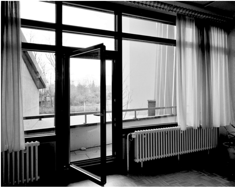
Figure 38: St. Maria, Ditzingen, meeting room. Photo by the author.
