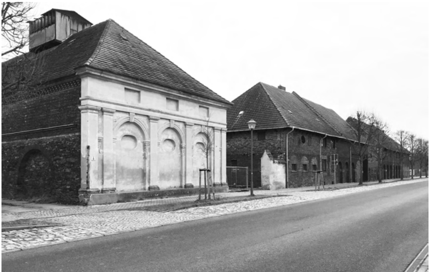
Fig. 11.5: Amtshaus of Wörlitz, rear farmyard, wings at the country road (photo: Günther).
