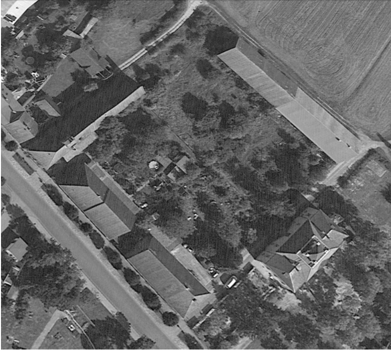
Fig. 11.11: Amtshaus of Wörlitz with rear farm yard (photo: GoogleEarth).
