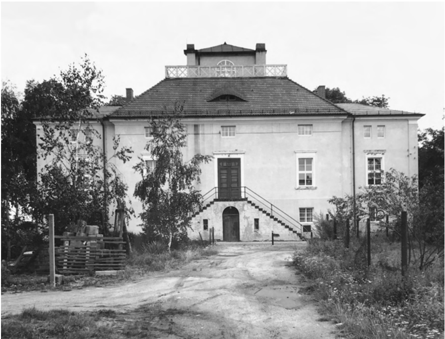
Fig. 11.10: Amtshaus of Wörlitz, rear side, present state, the staircase added later (photo: Günther).
