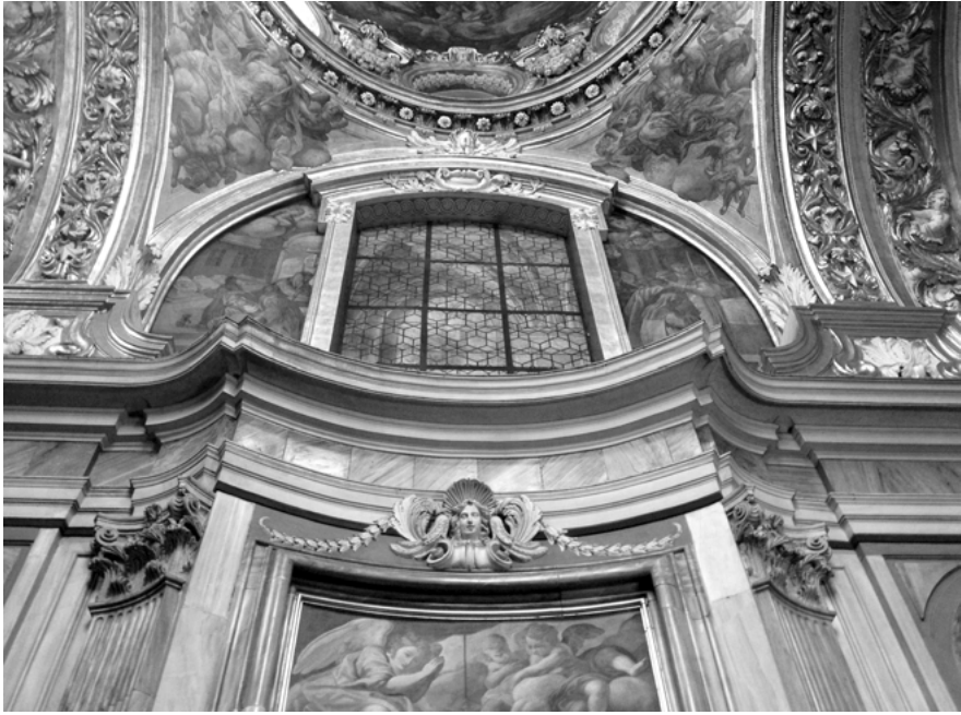
Fig. 12.13: Wrocław, Cathedral St. Elizabeth's Chapel, concave prominence of side walls (photo: Andreas Nierhaus, Vienna).
