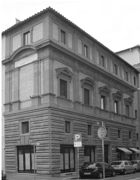
Fig. 9.15: Palazzo Jacopo da Brescia (photo: author). The original palace, on a site on the Borgo Nuovo close to St Peter's, was demolished in 1936 but then rebuilt nearby on the Via Rusticucci.
