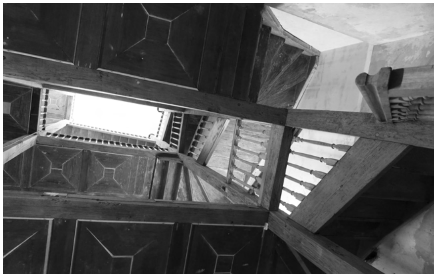
Fig. 11.14: Amtshaus of Wörlitz, stairwell, during restoration (photo: Günther).
