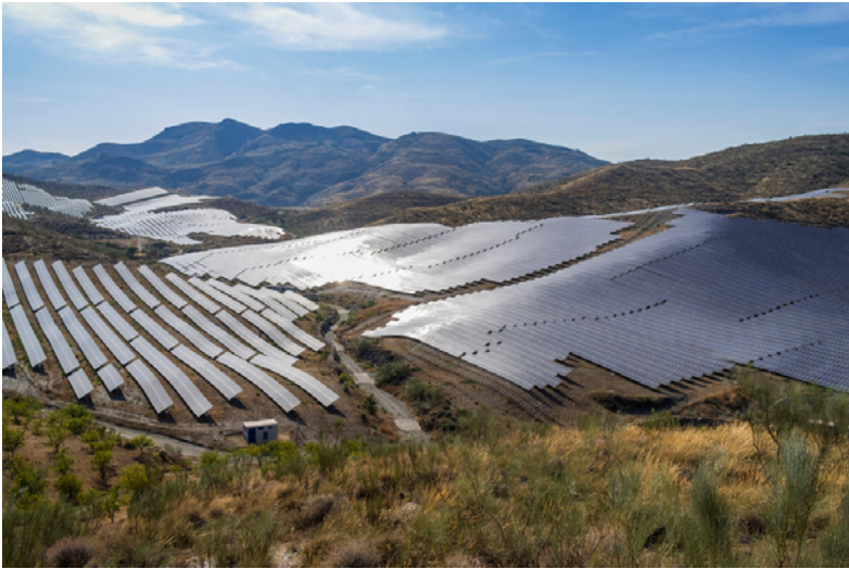
FIGURE 11.2 Lucainena de Las Torres 2 photovoltaic power station covering valleys and hillsides in Andalucía, 2013 SOURCE: ANDREW WATSON/CLIMATE VISUALS COUNTDOWN, HTTPS://CLIMATEVISUALS.ORG/ASSET/2552/
