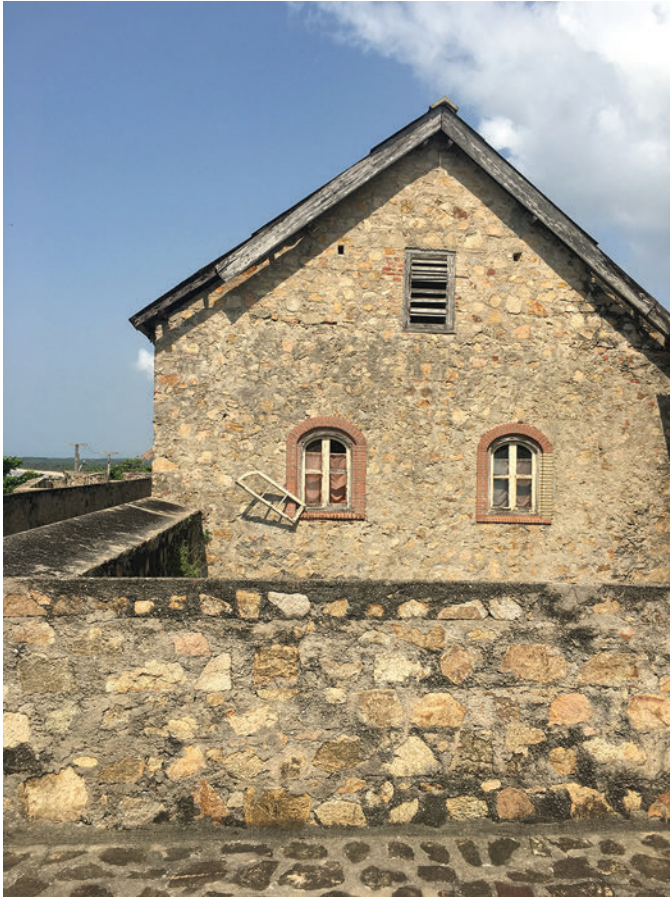
Figure 3. Exterior wall of Groß-Friedrichsburg, built in 1683, in 2020, Princes Town, Ghana. (Photo by the author.)
