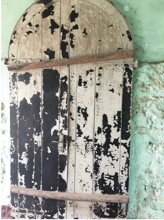
Figure 9. Exterior door, German colonial station, Kpando. (Photo by the author.)
