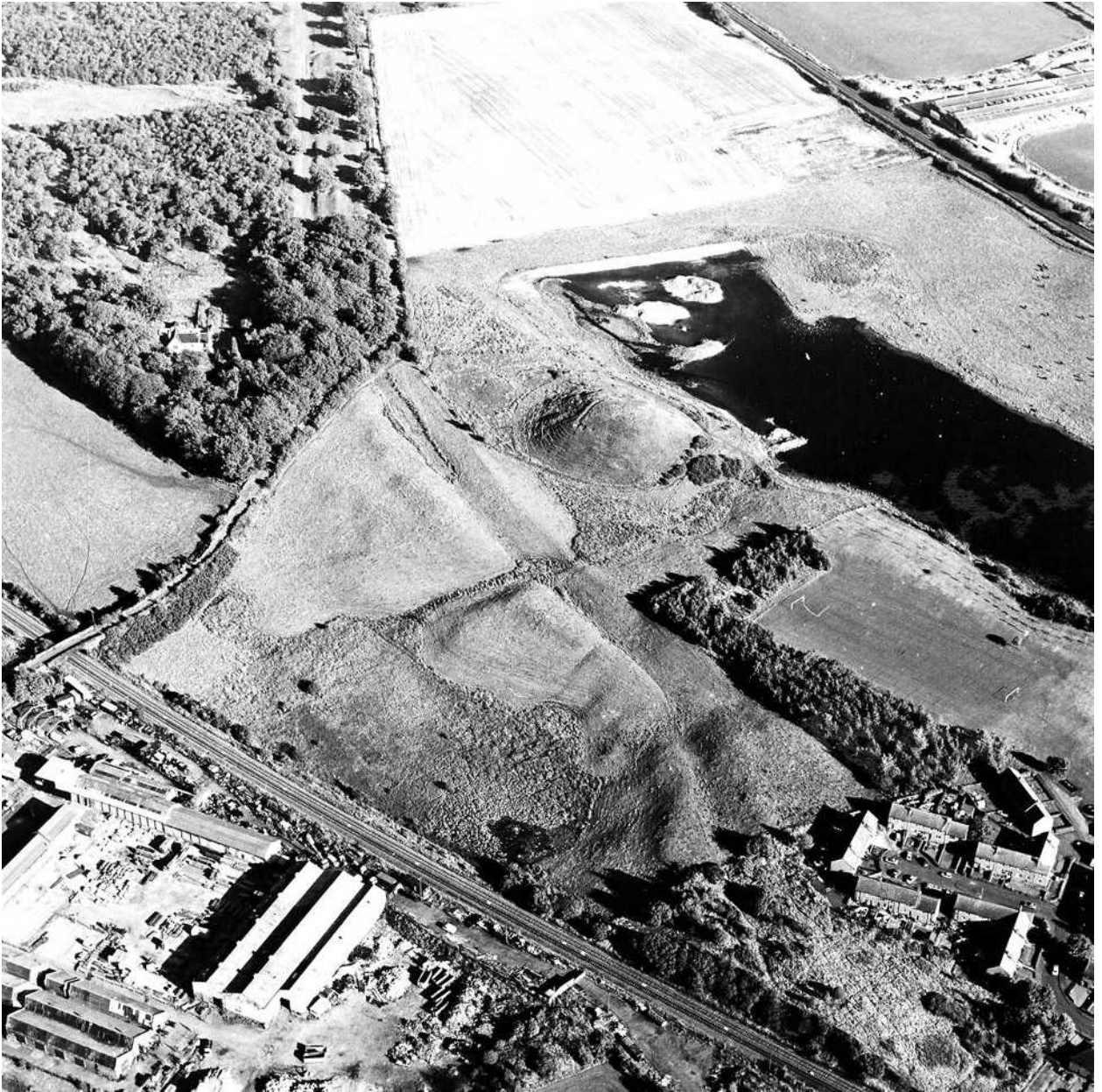
Figure 6.1.2. Aerial photograph of the extant line of the Ditch and Upcast Mound at Bonnyside from the west. Elf Hill lies to the south of the Wall in the centre of the image, with the line of the Military Way running between it and St. Helen's loch (© Historic Environment Scotland SC 1725941).
