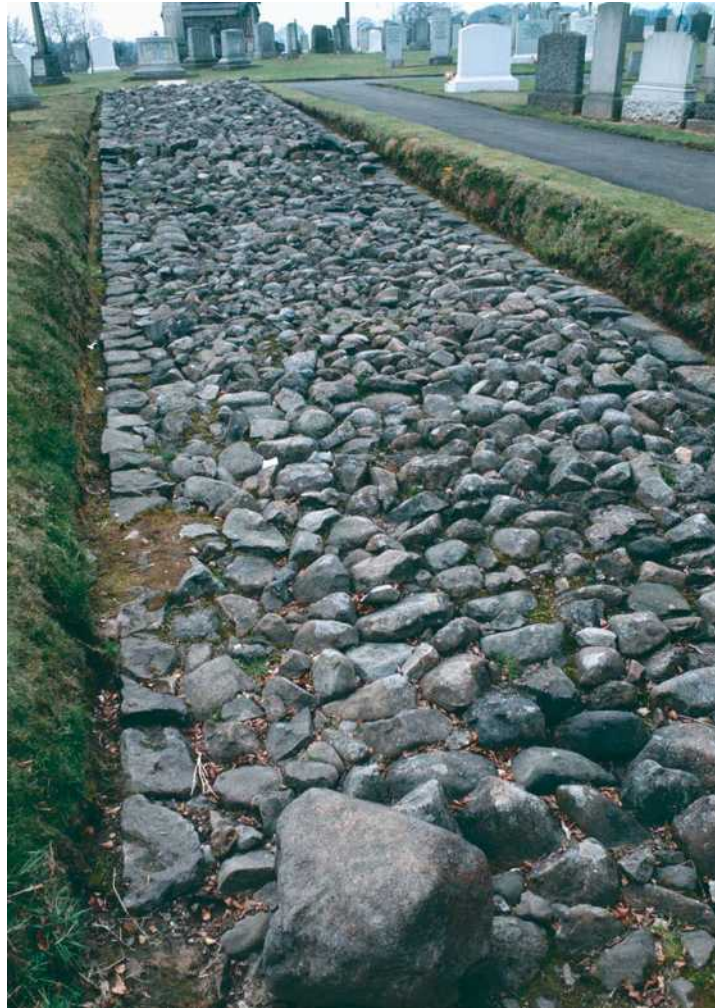
Figure 1.17. Extant remains of the Rampart base and a culvert in New Kilpatrick cemetery. View from the east.
