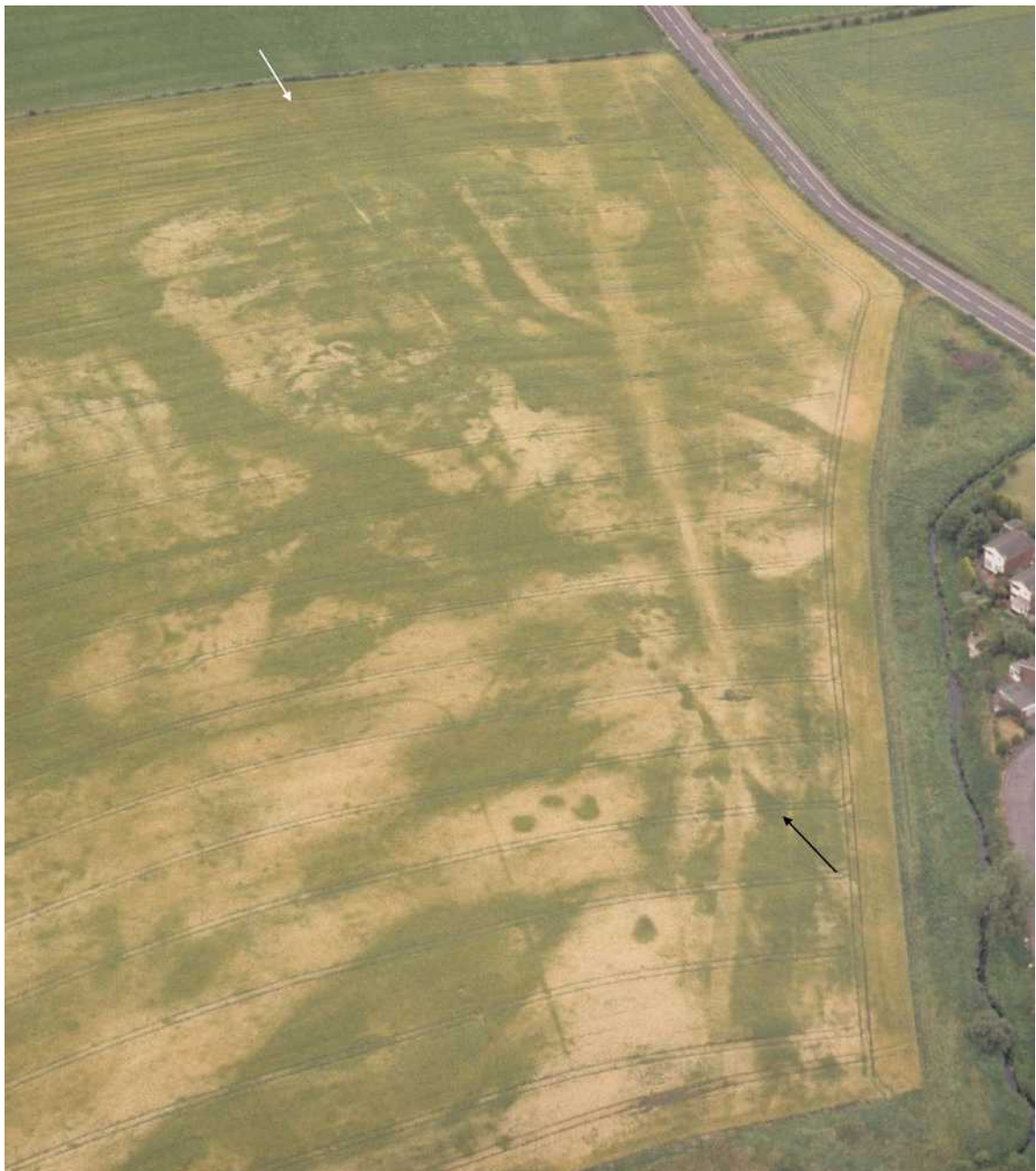
Figure 1.8. Aerial photograph of part of the camp at Easter Cadder (left foreground) with the line of the Antonine Wall Ditch, Rampart (arrowed in white) and the Military Way (arrowed in black) beyond it to the right, all bisected by a modern pipeline. All are revealed as cropmarks, the Military Way primarily as a line of quarry pits. View from the east.
