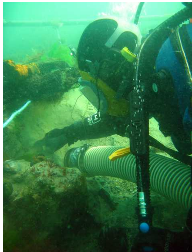
Figure 2.5. Diver excavating with dredge
