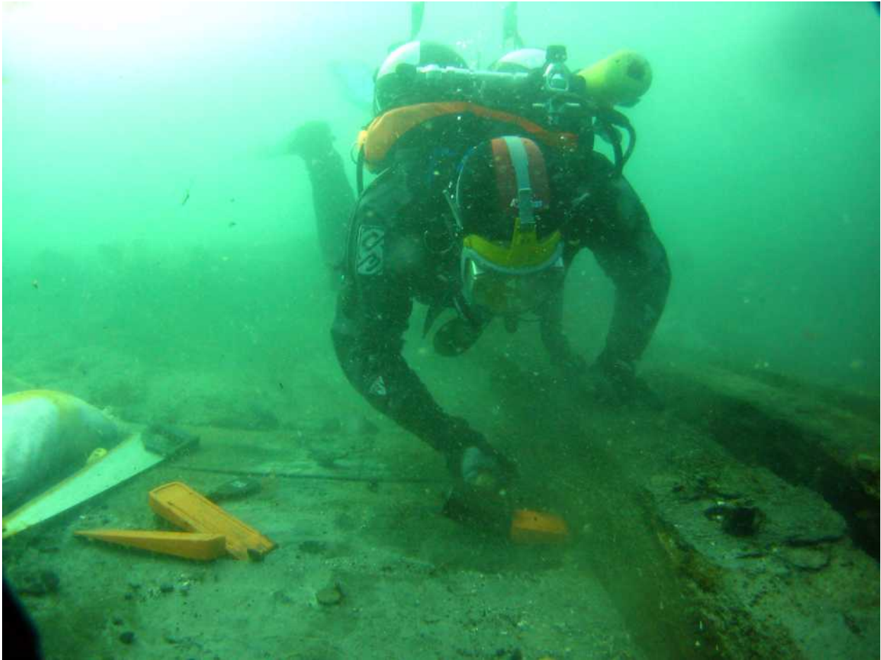
Figure 2.9. Dismantling the timbers underwater
