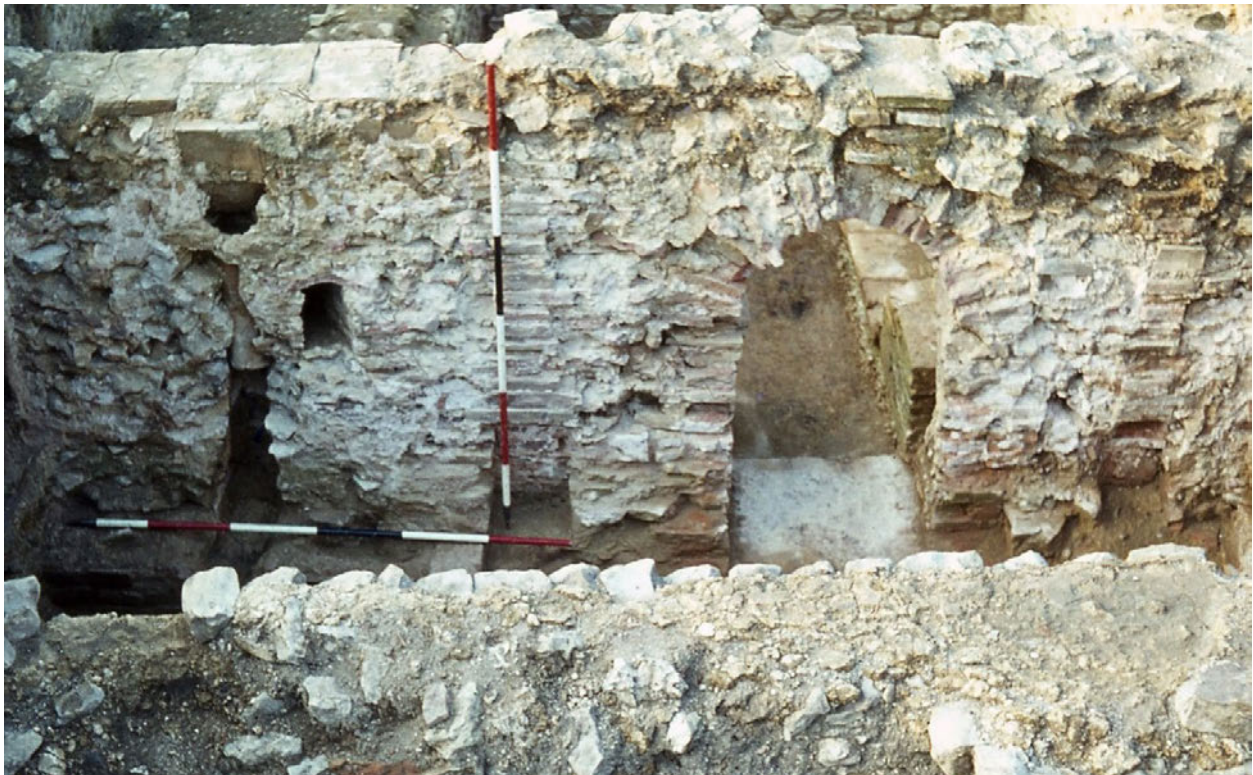
Figure 3.17. Same view with opus signinum removed to reveal furnace arch (unblocked), drain and wall flues of Period 2A (Room 58).
