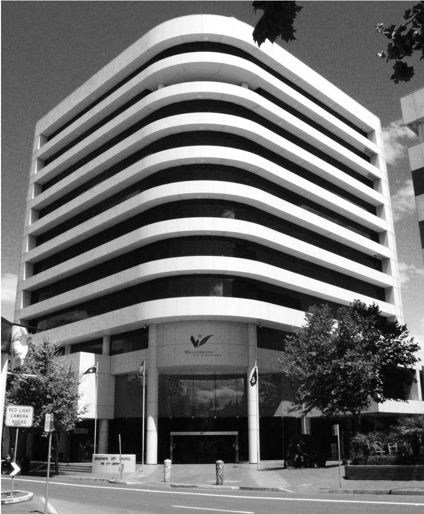
Plate 7.2 The Wollongong City Council administration building, completed in 1988, photographed in 2008
