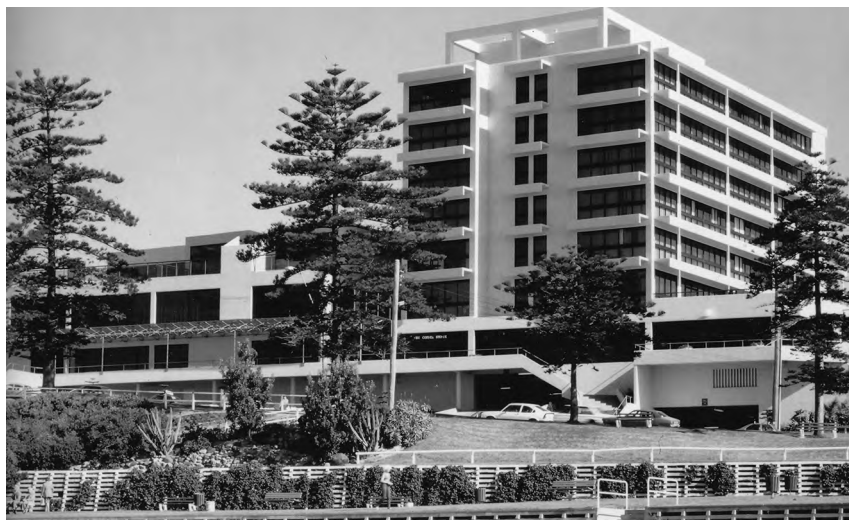
Plate 5.1 The North Beach International Hotel in North Wollongong, photographed from the beach, 17 November 1988
