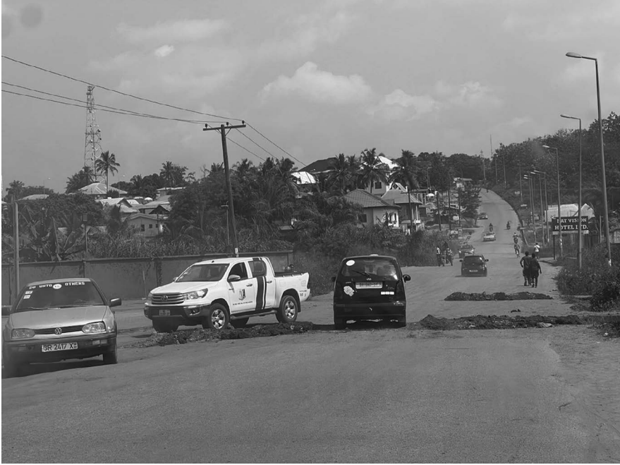
Figure 5.1 Auto-constructed speed bumps
