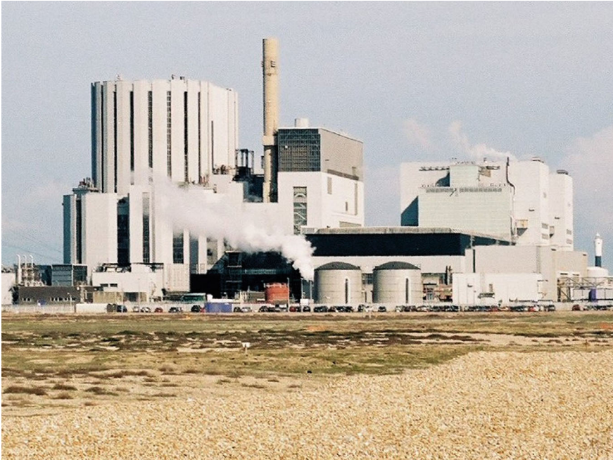
Fig. 4.1 Dungeness B AGR Nuclear Power Station. Image source public domain via Wikimedia Commons (Sandpiper)
