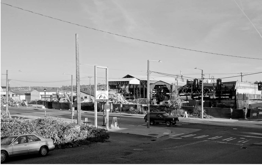
Figure 4.1 National Nordic Museum construction site in Ballard.
