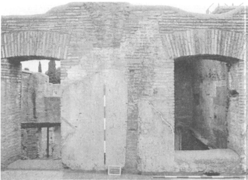
Figure 5.7 Marks of curtain wall in Rm 129.
