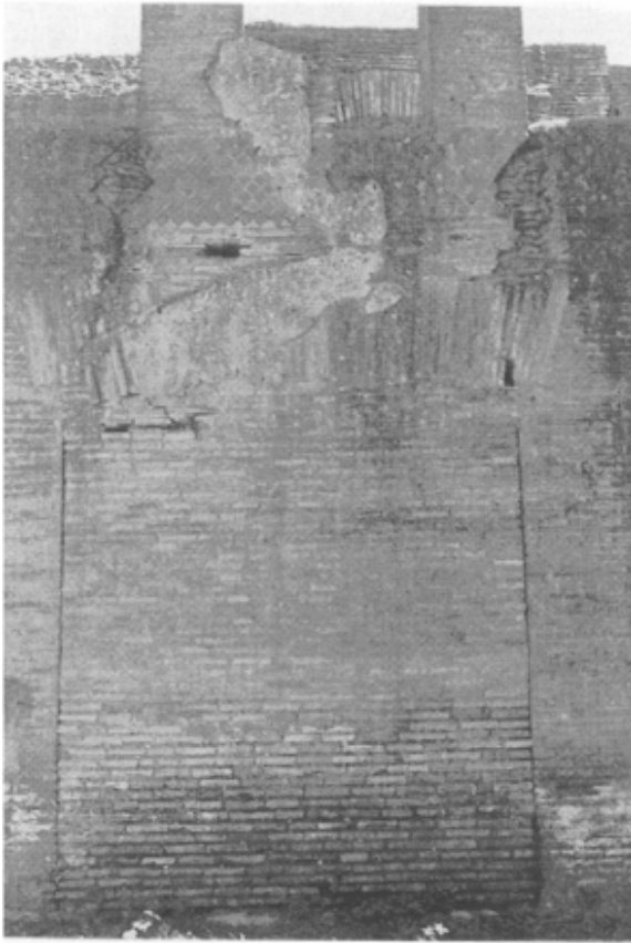
Figure 5. 6 Blocking of opening Rms 26/29.
