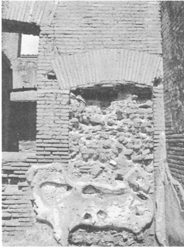
Figure 5.5 RMs 24/25, blocked doorway.
