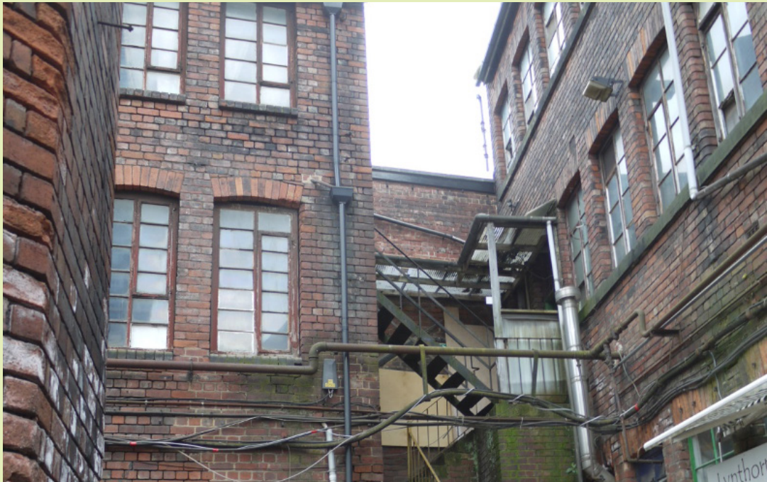
FIGURE III.3.3 Portland Works – Internal Courtyard. Photo by Mark Parsons.
