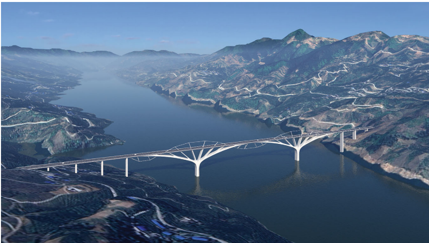
Fig. 7.3 Rendering of a long-span steel–concrete composite bridge, optimized using a multi-material BESO method (reprinted from Li et al. 2022, with permission from Elsevier)
