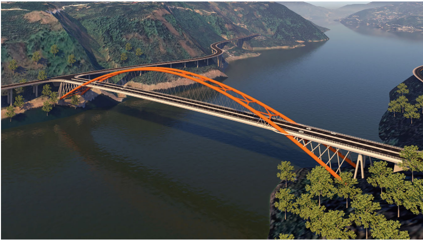
Fig. 7.2 Rendering of the Kui Zhou Yangtze River Bridge, with its wind bracings and arch bearings optimized using the BESO method (reprinted from Lai et al. 2023, with permission from Elsevier)
