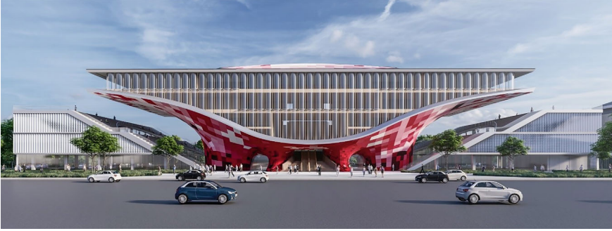
Fig. 7.1 Rendering of a five-storey architectural complex named ‘Xiong’an Wings’, with its core structural system optimized using the BESO method. Construction completed in 2024 (reprinted from Li et al. 2023, licensed under CC-BY 4.0)
