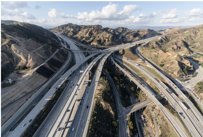
FIGURE 6. Looking north at the Newhall Pass Interchange where the 5 and 14 highways merge. The 14 splits to the right, heading northeast towards the Antelope Valley. Source: trekandphoto, Adobe Stock.
